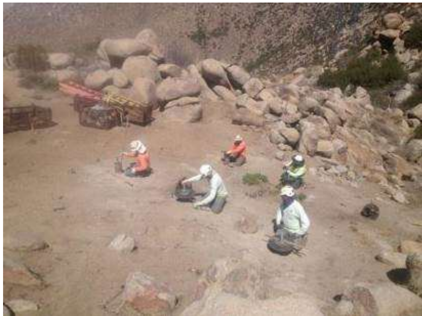
Figure 4. Permanent platform installation activities at Tower 1045 (Photo courtesy of FRED).
