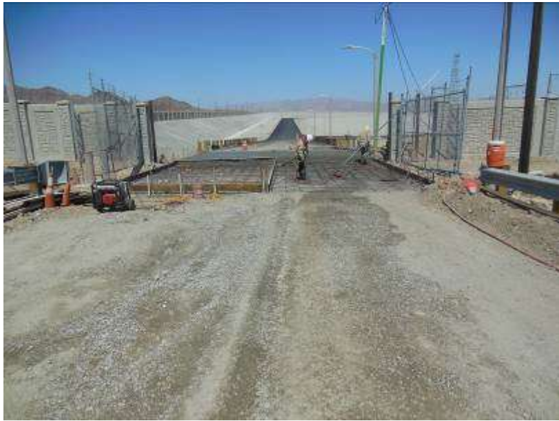
Figure 9. Setting forms and pouring concrete at the Red Bluff Substation entrance.
