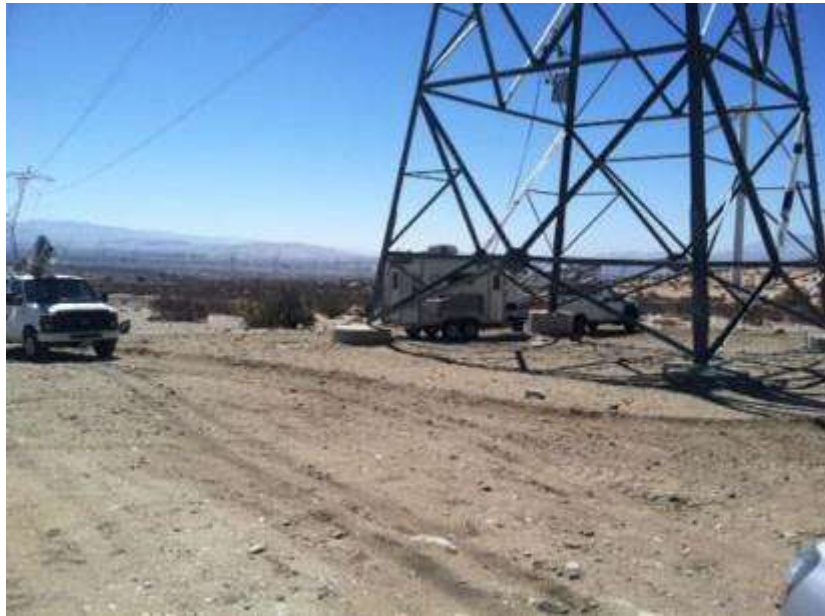
Figure 3. Telecomm splicing activities at Tower 1010.
