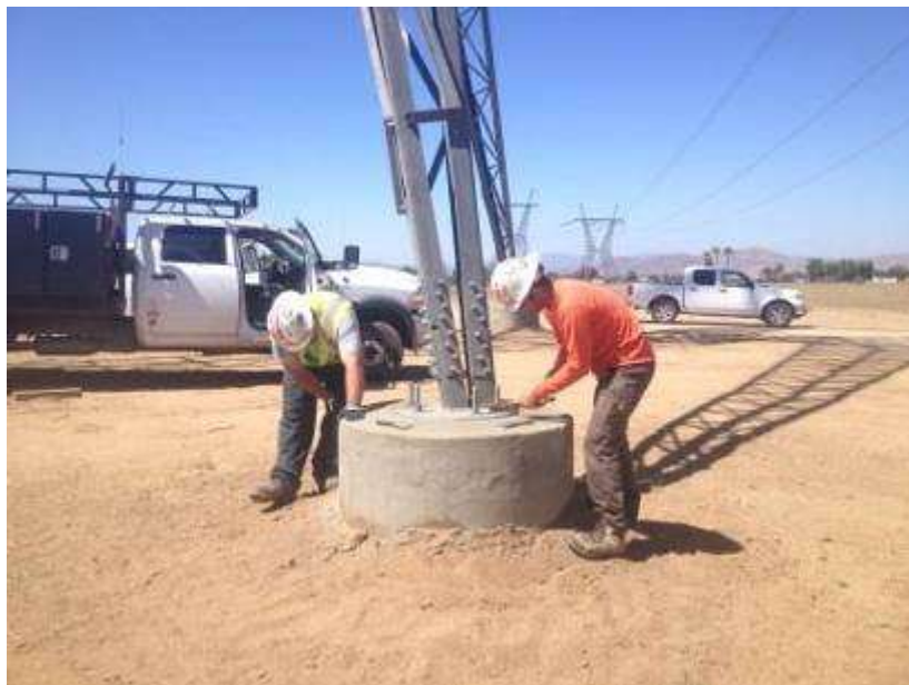
Figure 2. Low-intensity QA/QC activities (leg painting) at Tower 1152.
