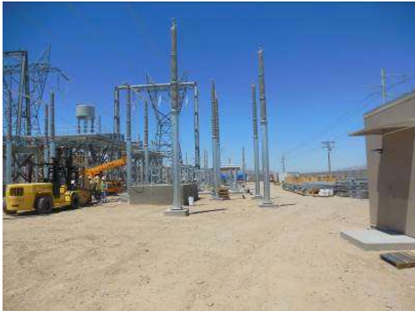
Figure 10. Construction activities at the Series Capacitor site.
