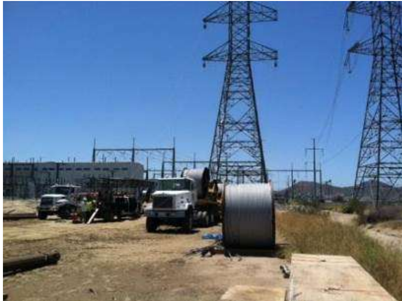
Figure 1. Wire pulling activities occurring at Pull Site 51 near Towers 1156 and 1157.
