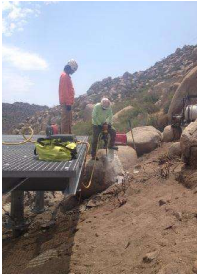
Figure 3. Permanent platform installation at Tower 1048 (Photo courtesy of FRED).
