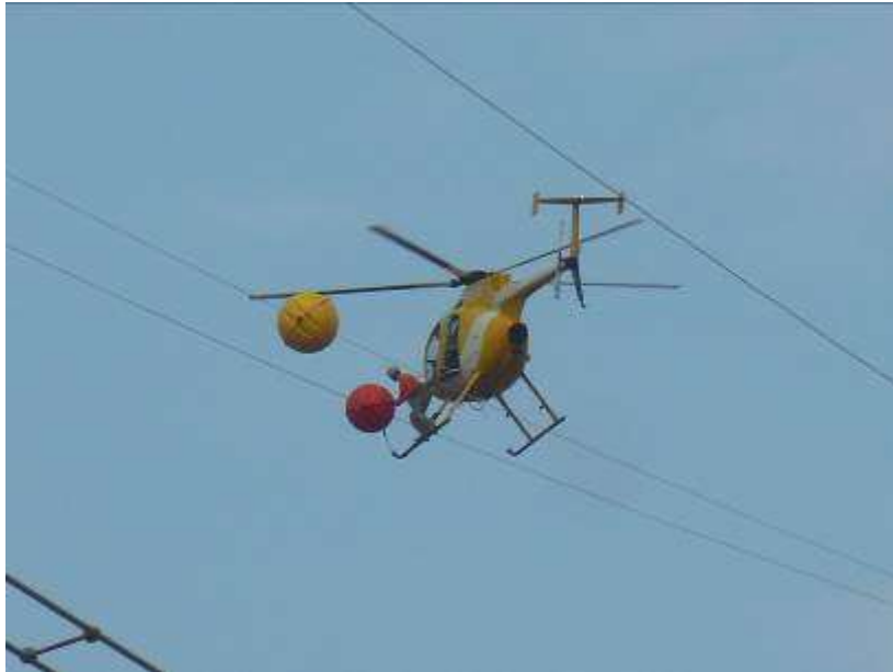
Figure 1. Marker ball installation between Towers 1090 and 1091.
