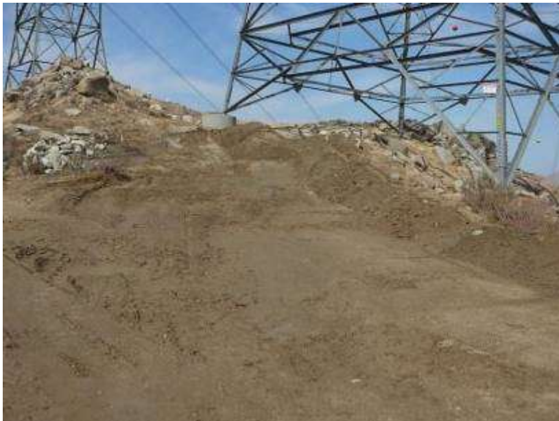
Figure 2. Site stabilization activities at Tower 1071 (Photo courtesy of FRED).
