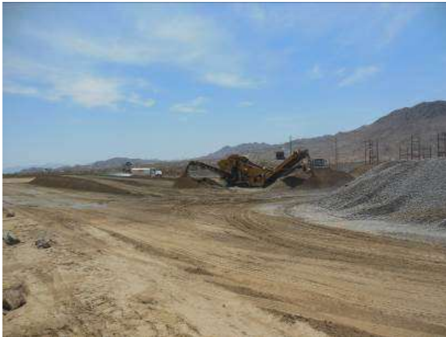
Figure 4. Removal and sorting of gravel at the Chiriaco Summit Yard.
