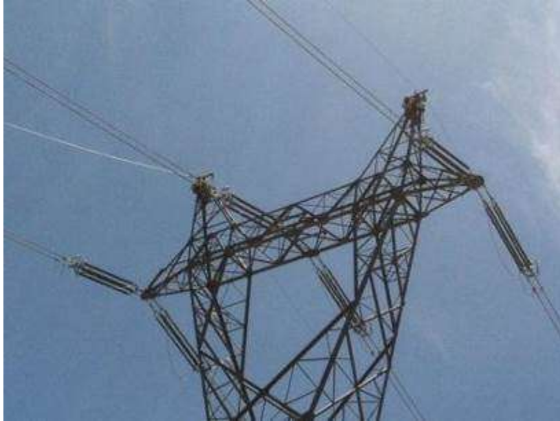
Figure 1. OPGW wire work at Tower 1106.
