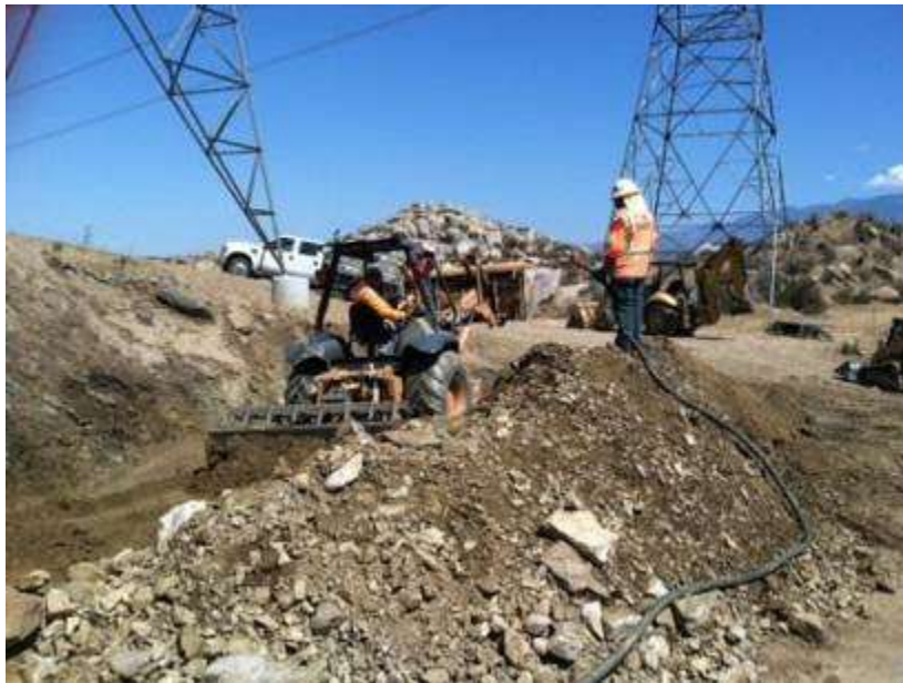
Figure 2. Site stabilization activities at Tower 1082.
