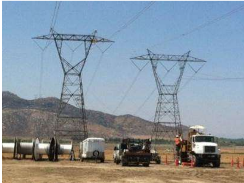
Figure 1. OPGW wire pull set-up at Tower 1116.
