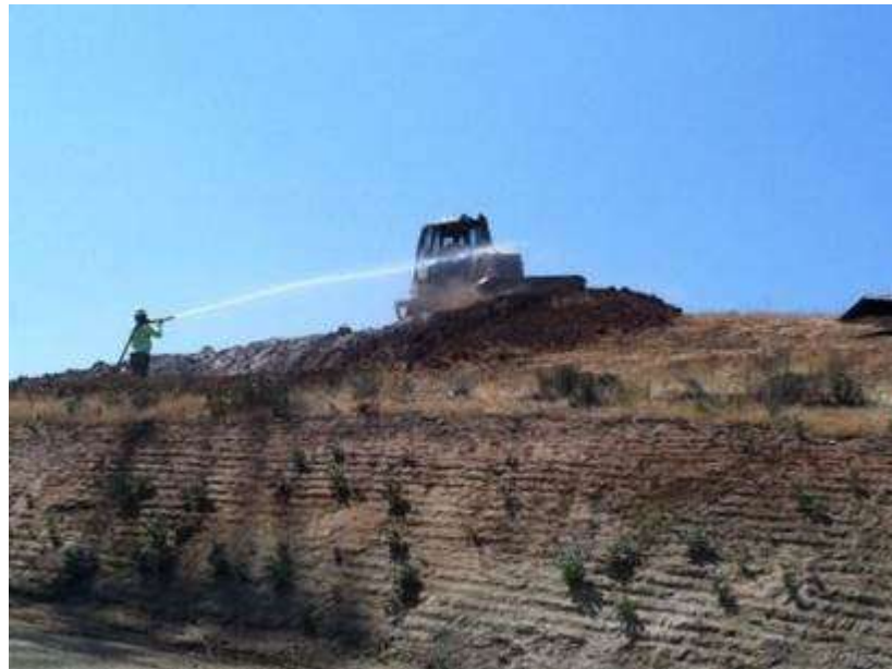
Figure 2. Site stabilization activities at Tower 1091.
