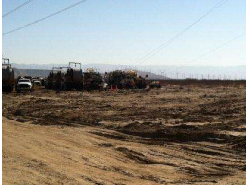
Figure 1. Wire stringing activities at Wire Site 10 (near Tower 1031).
