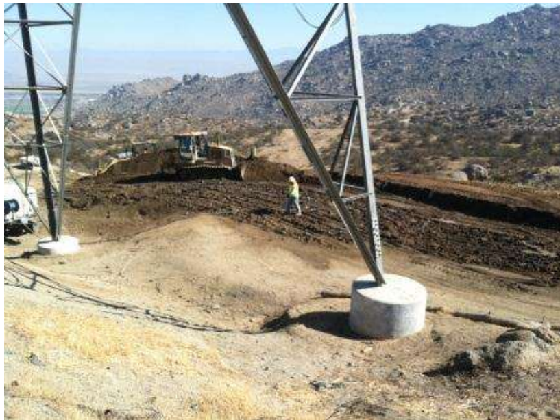
Figure 2. Site stabilization activities at Tower 1128.
