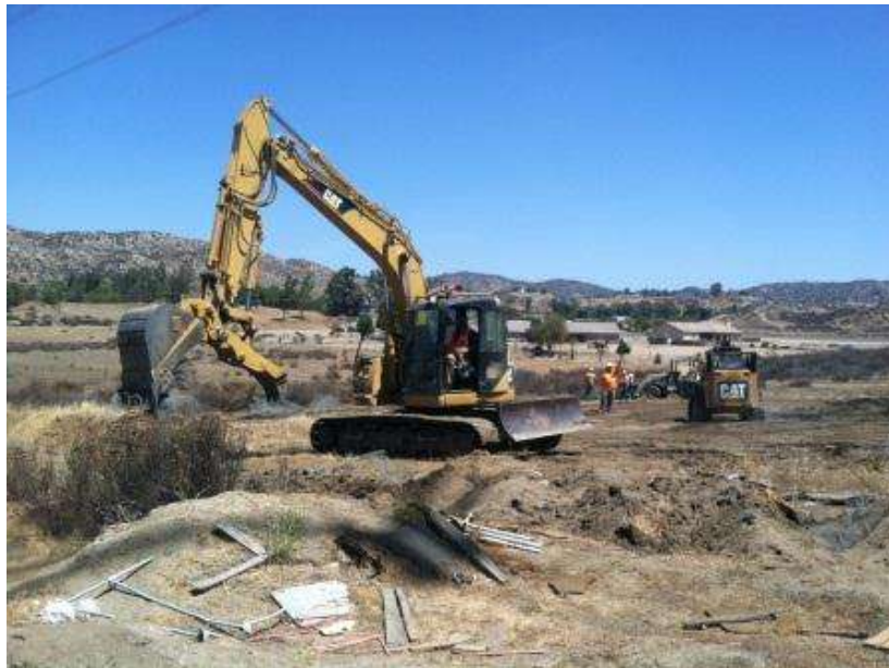
Figure 3. SKR fencing removal and site stabilization activities at Tower 1134.
