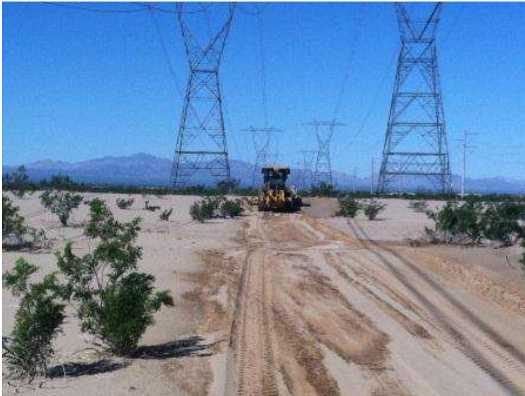
Figure 1. Maintenance grading of main access road near Tower 2636.
