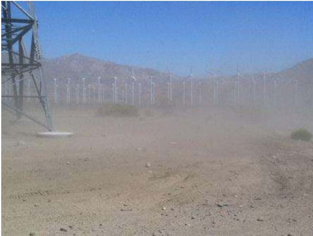
Figure 3. Excessive fugitive dust observed at HLZ H2.
