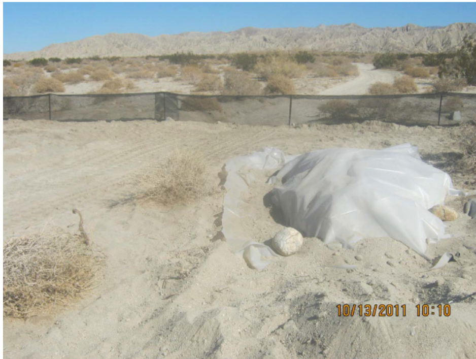
Figure 4: Contaminated soil from hydraulic fluid spill at Tower #2132 was isolated in plastic sheeting and removed from site the following day.
