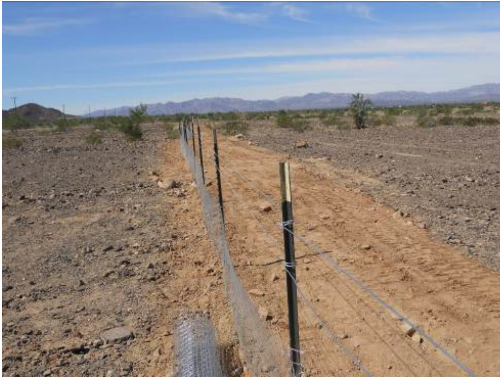
Figure 8: Exclusionary fencing activities completed at the Red Bluff Substation site. Note top wire along fence to prohibit bighorn sheep entry.
