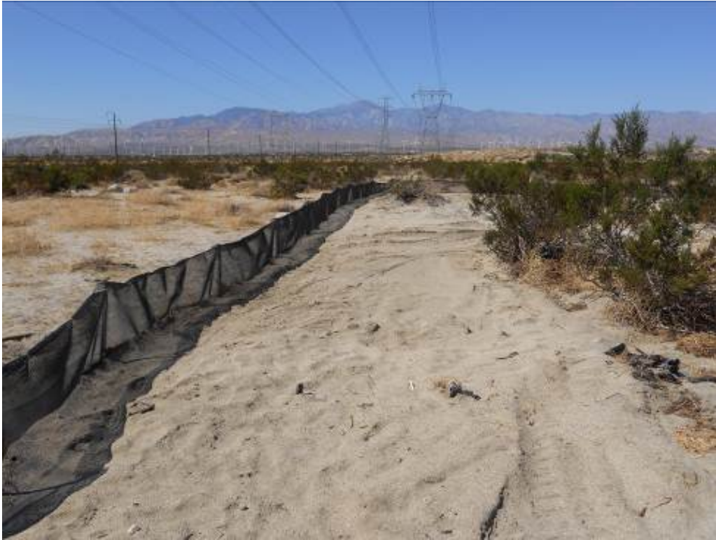
Figure 1: Completion of exclusionary fencing activities at one of the tower locations.
