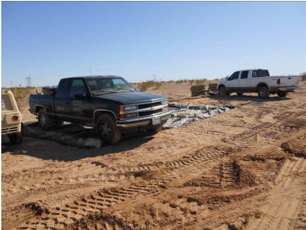
Figure 7: BMPs implemented, including contained parking areas, at the CRS site.
