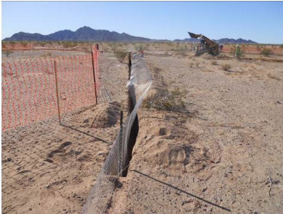
Figure 6: Installation of desert tortoise exclusionary fencing at CRS site.
