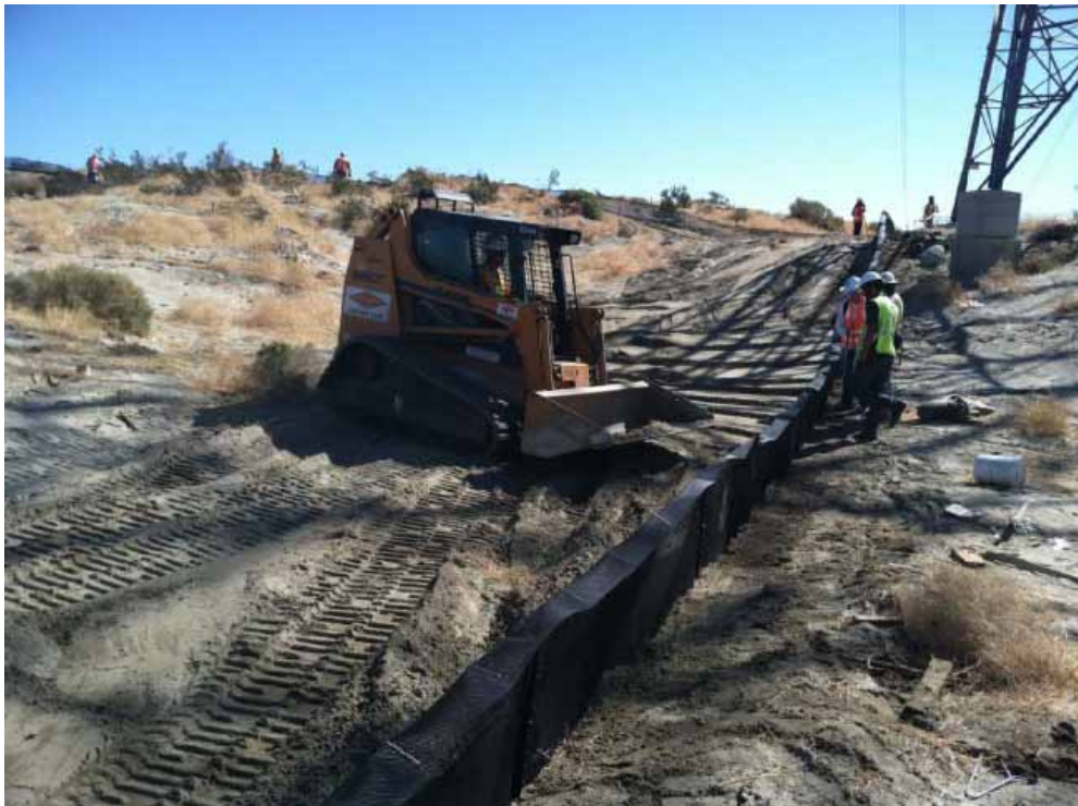
Figure 2: Backfilling of trench at Tower #2013 during exclusionary fencing activities.
