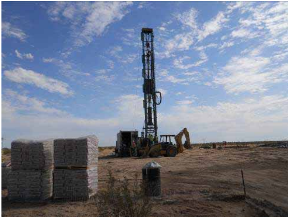
Figure 5: Erection of drill rig at CRS.
