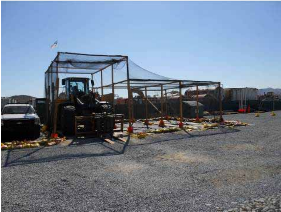
Figure 1: Bird netting and BMPs effectively installed at Meniffee Construction Yard.
