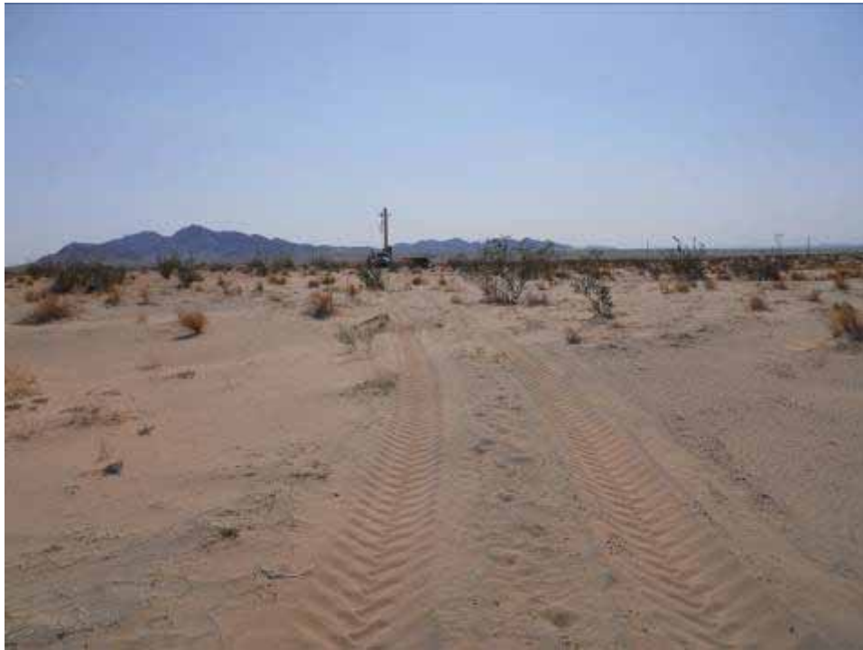
Figure 3: View south along “drive and crush” road created for Red Bluff distribution line.
