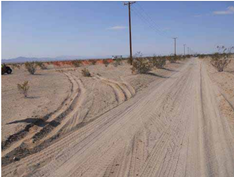
Figure 5: Vehicle tracks outside of disturbance limits along the Red Bluff distribution line access route. This incident resulted in the issuance of a Project Memorandum from the CPUC EM.
