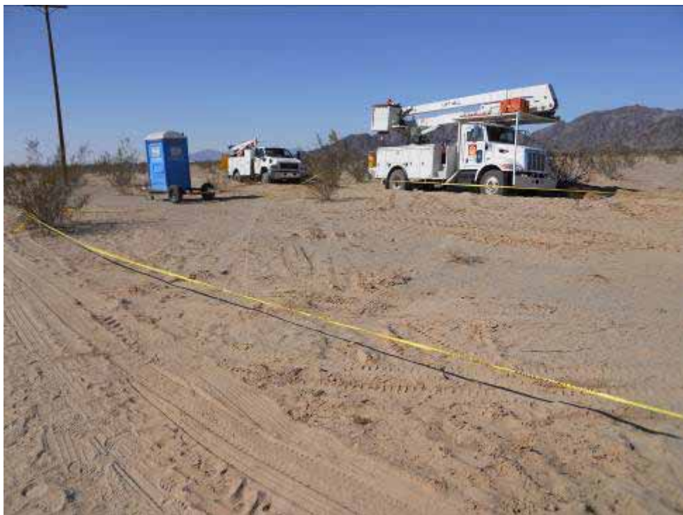
Figure 6: Area outside of approved Red Bluff disturbance limits which was repeatedly crossed by construction vehicles. The SCE Biological Monitor placed yellow caution tape around perimeter for future avoidance.
