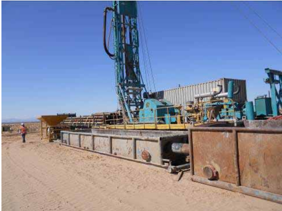
Figure 8: Drill rig assembly being conducted at CRS.
