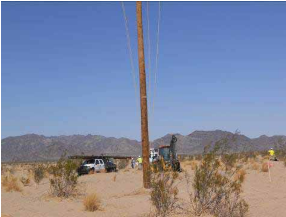
Figure 4: New pole installation along the Red Bluff distribution line.
