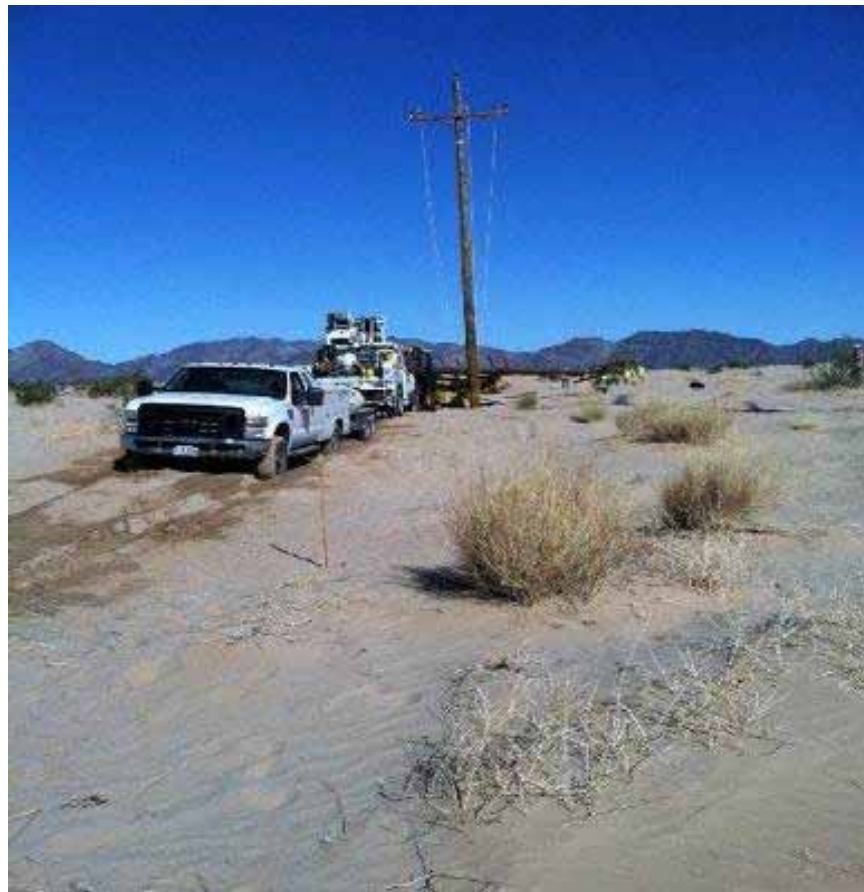
Figure 5: Installation of wooden poles along the CRS distribution line.
