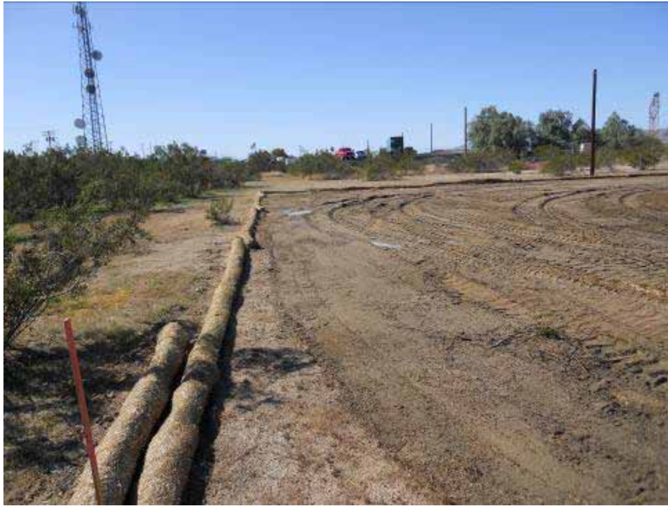
Figure 1: Installation of BMPs and grading at the Summit Construction Yard.
