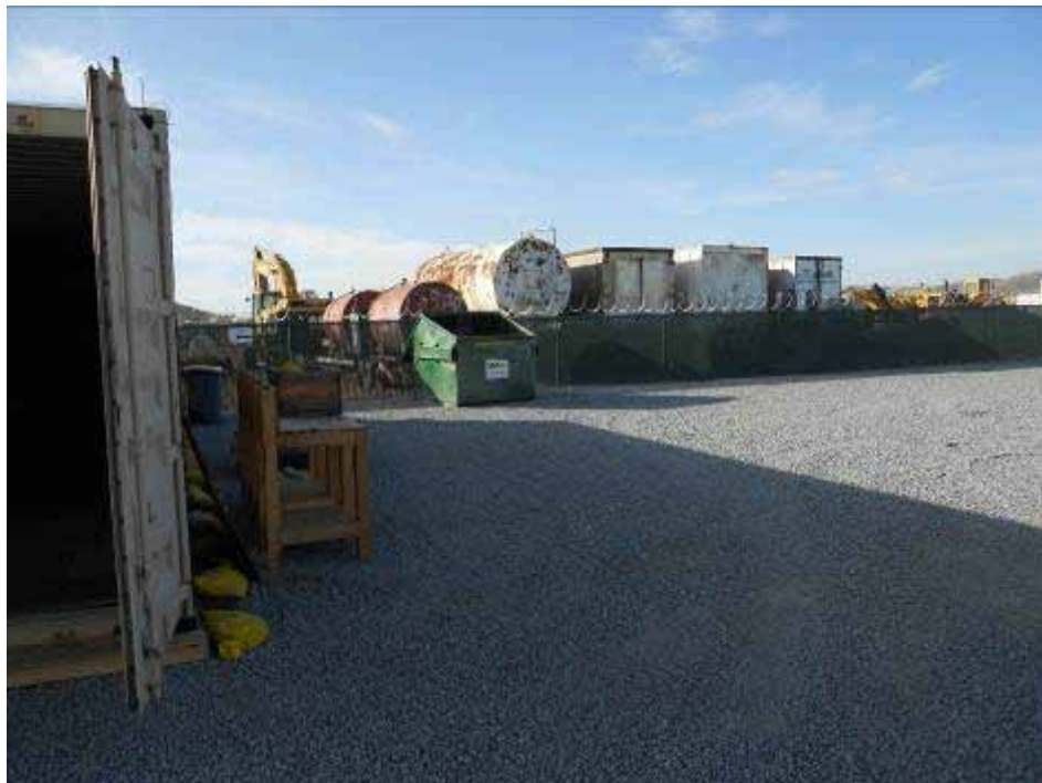
Figure 4: Open trash container at the Meniffee Construction Yard. The Kenney site representative was made aware by the CPUC EM and immediately closed the container.
