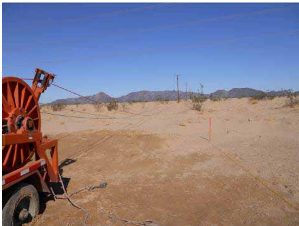
Figure 6: Wire stringing activities occurring along the CRS distribution line.
