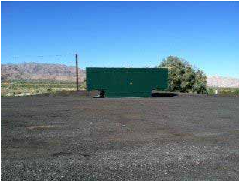
Figure 2: Water tank located in barren lot adjacent to western boundary of the Summit Construction Yard. This area was outside of the approved disturbance limits and the tank was relocated the following day.
