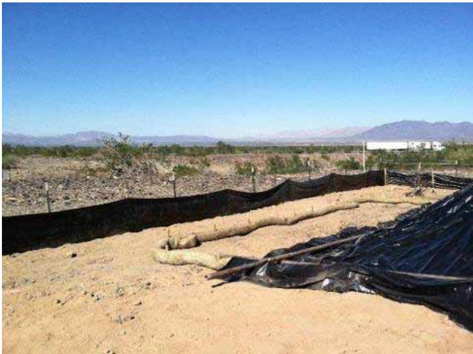
Figure 8: Silt fence installation around Red Bluff drill site.
