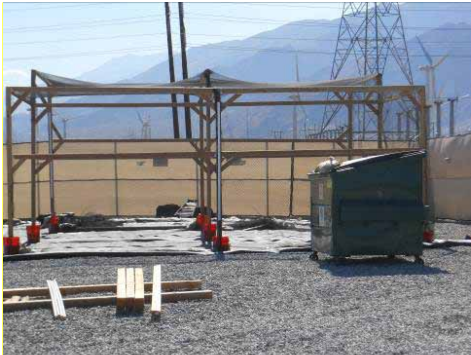
Figure 2: Netted equipment port constructed at Devers Construction Yard to limit impacts from nesting birds.
