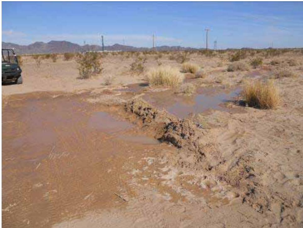
Figure 4: Location of check dam at CRS that was breached by surface flows resulting from well water release (reported as a Level 1 non-compliance incident by SCE).
