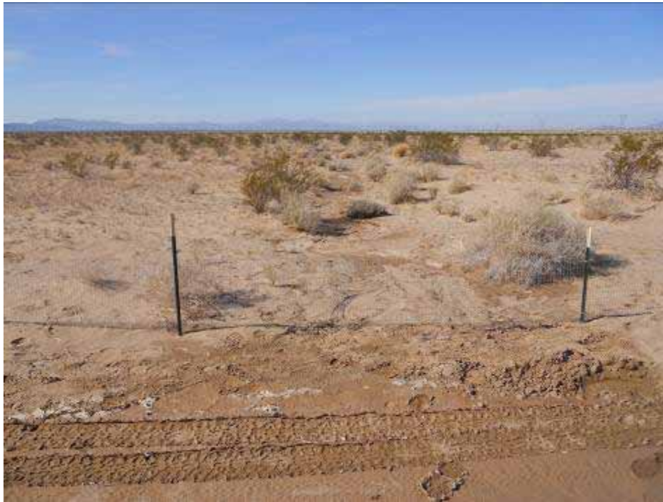
Figure 5: View west towards area where surface flows from well release had flowed outside of CRS disturbance boundaries. Note moist soils that were identified to approximately 200 feet downstream of this location.
