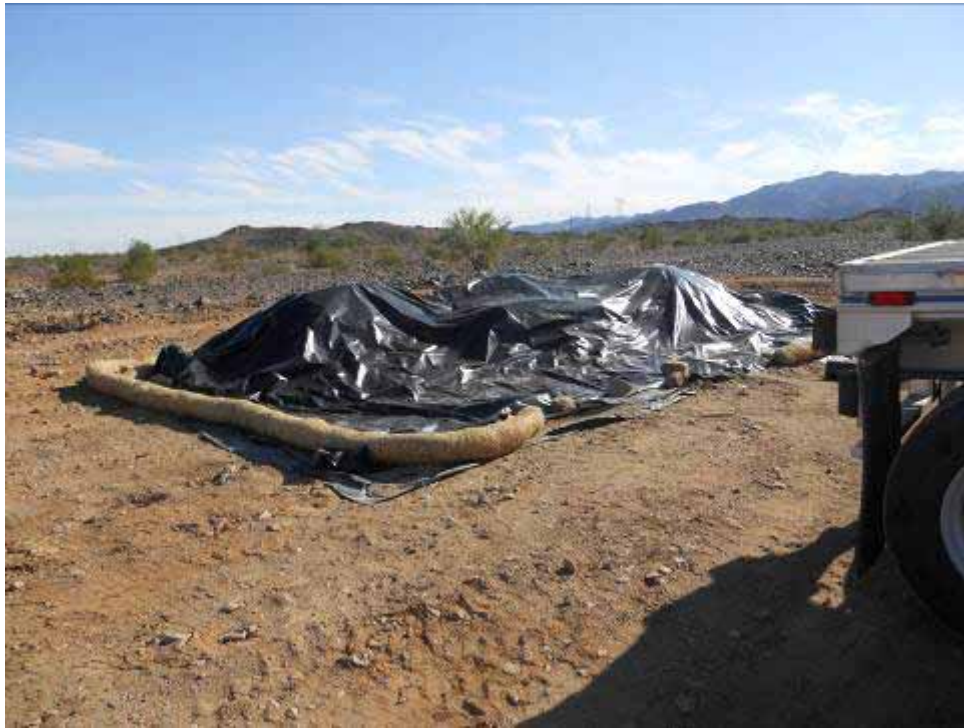
Figure 7: Containment of drill tailings at Red Bluff Substation.
