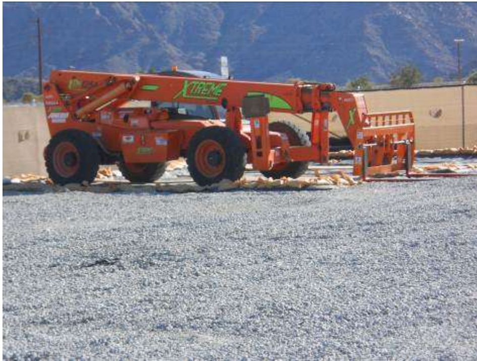
Figure 3: Heavy equipment parked on plastic sheeting at the Desert Center #2 Construction Yard.
