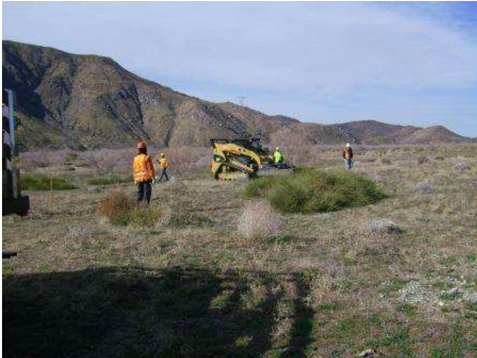
Figure 1. Vegetation clearing at Tower 1062/R2.
