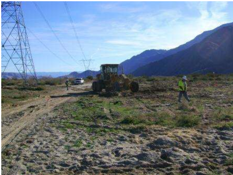
Figure 2. Grading at Tower 1064.
