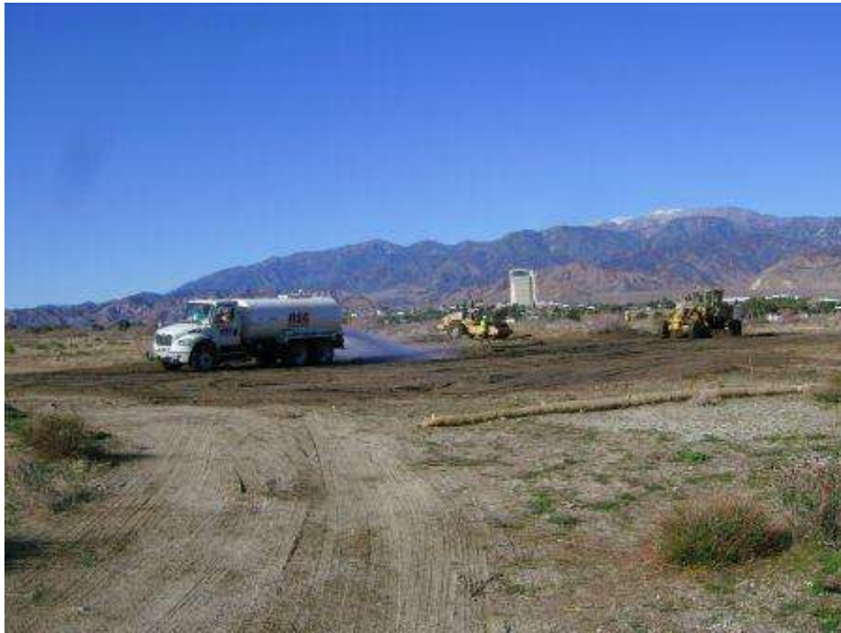
Figure 3. Fugitive dust control at Tower 1062/R2 during grading.
