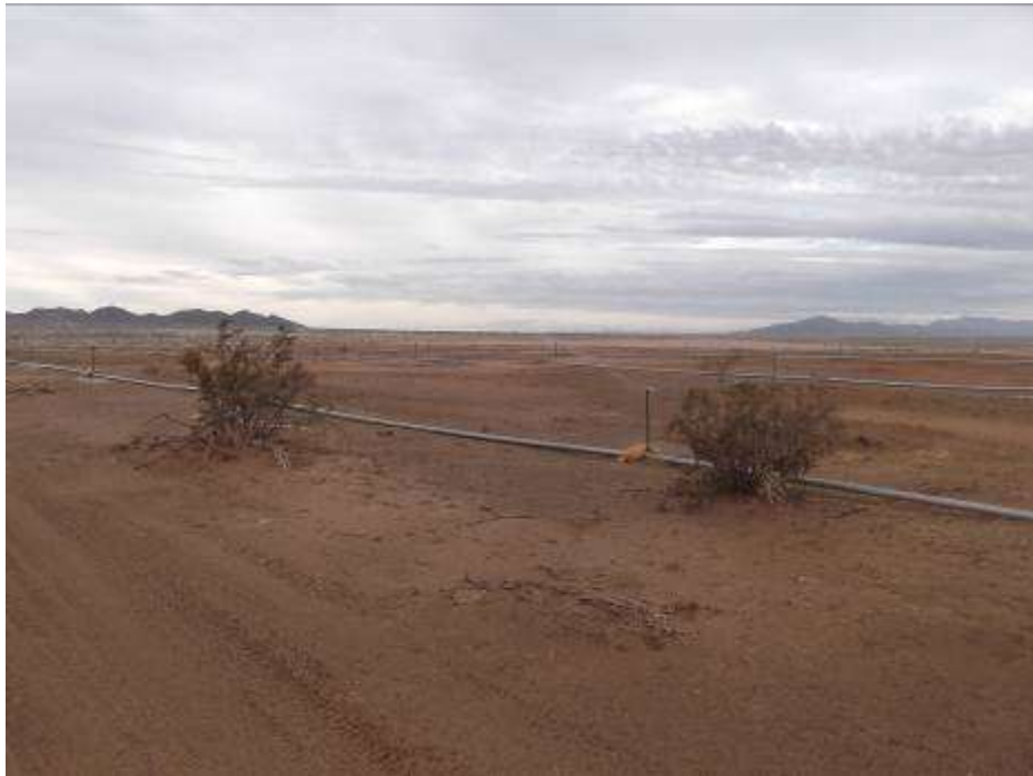
Figure 5. Sprinkler system installed at CRS to control water release from active well.
