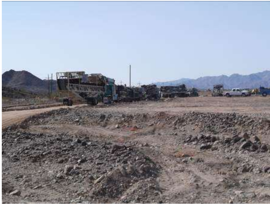
Figure 5. Rock crushing equipment being delivered to the Red Bluff Substation site.
