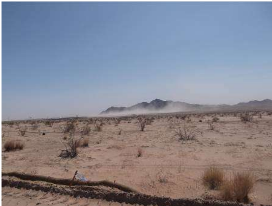
Figure 6. View southeast towards CRS from primary access road. Note excessive fugitive dust escaping project site.
