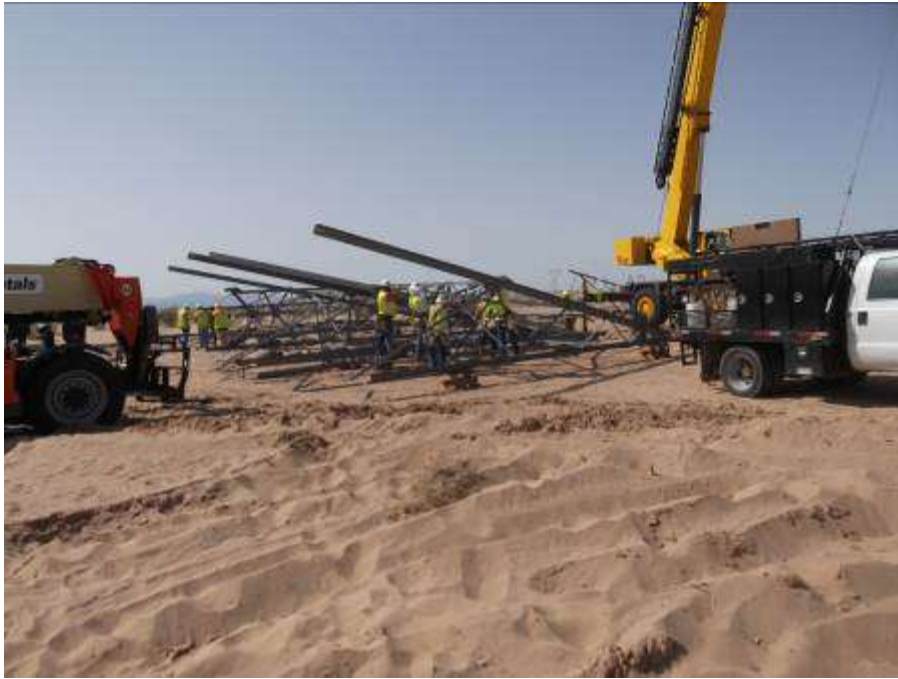
Figure 1. Tower assembly activities at Tower CR1-2W.
