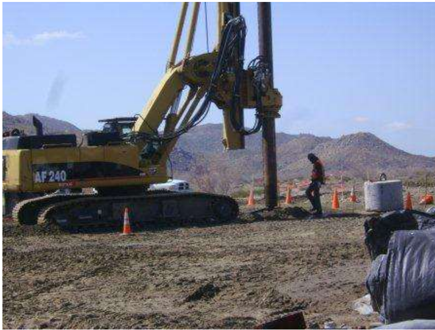
Figure 3. Foundation drilling at Tower 1062.
