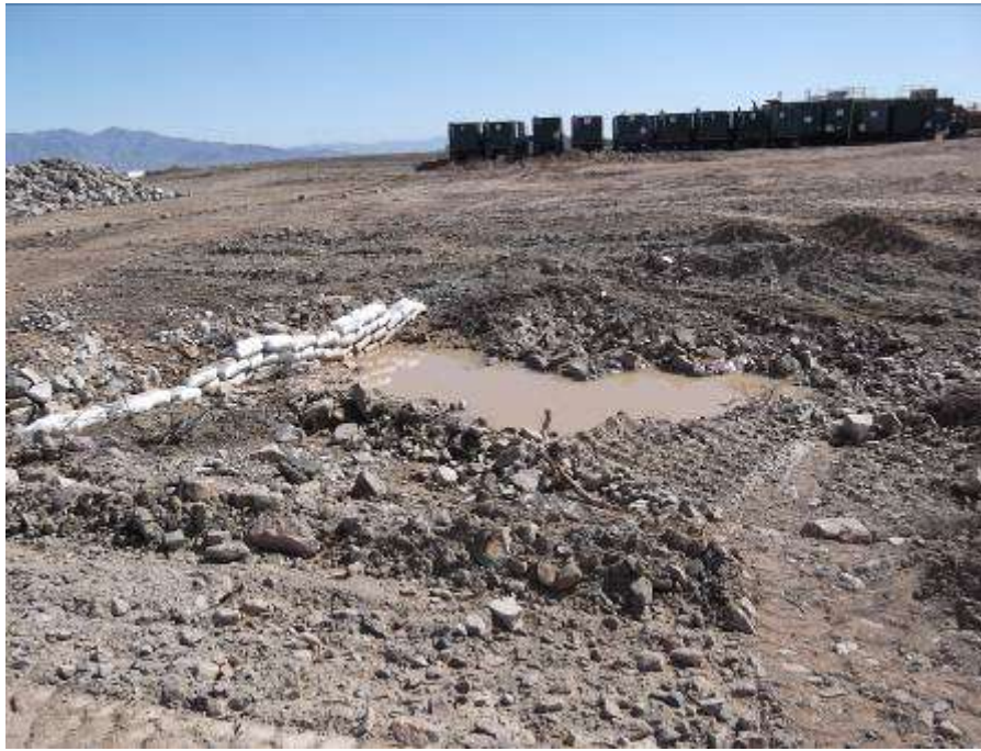
Figure 9. Water pooling behind check dam at Red Bluff Substation site.
