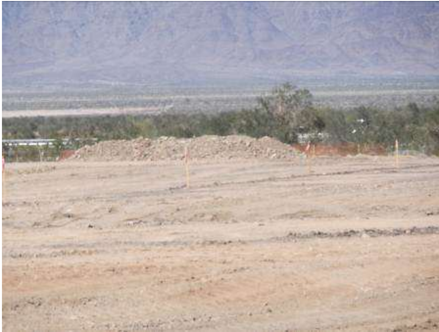
Figure 8. Desert pavement soils being stockpiled at Red Bluff Substation site.
