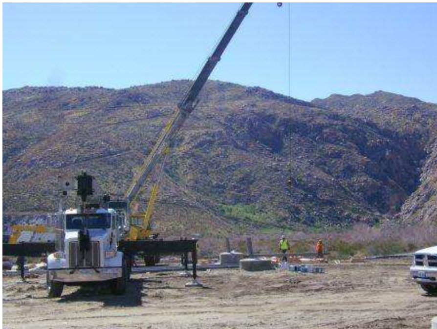
Figure 4. Crews begin tower assembly at Tower 1061.
