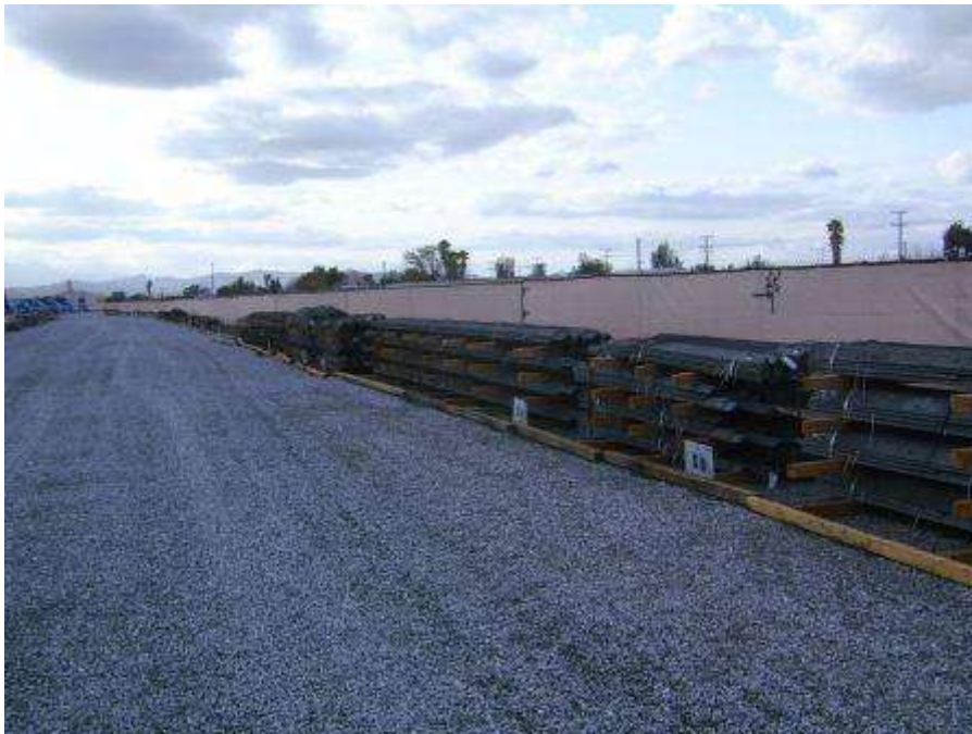
Figure 10. Materials at the Meniffee Yard covered with bird netting. The gravel shows sign of being dragged.
