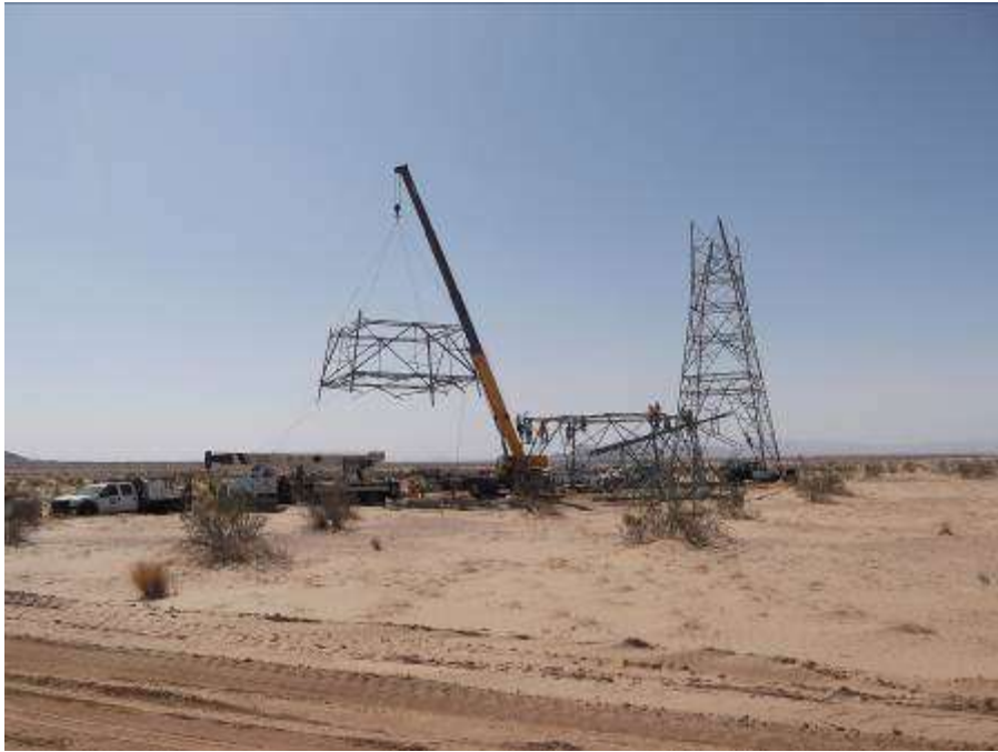
Figure 1. Tower assembly and erection activities at Towers 2649 and CR1-2W.
