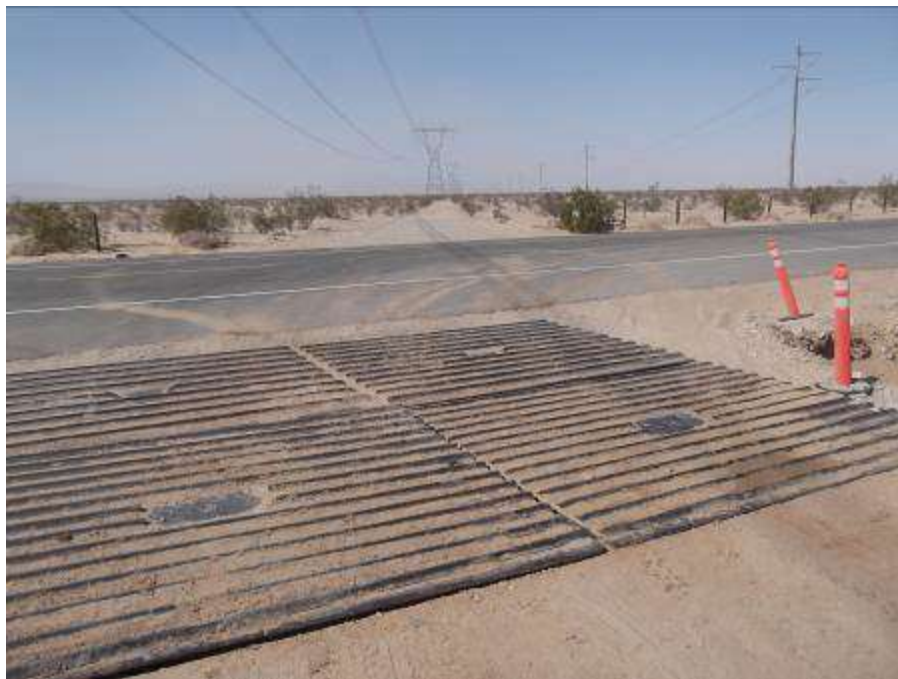
Figure 8. Excessive track-out observed by CPUC EM at ingress/egress to CRS primary access road.
