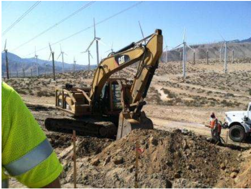
Figure 3. Spur road and crane pad grading at Tower 1014
