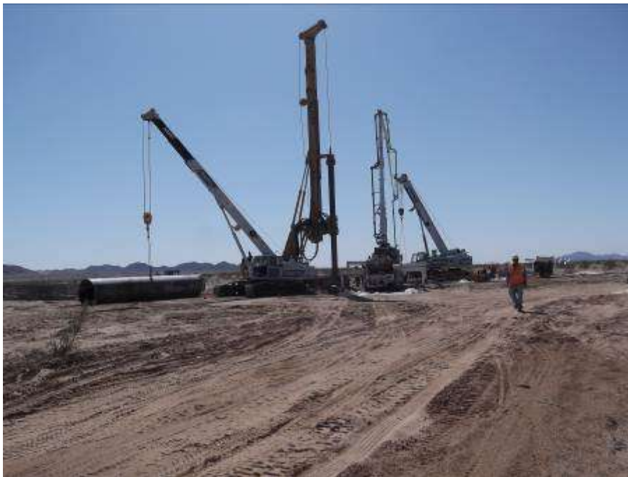
Figure 2. Foundation drilling at Tower CR1-2E.
