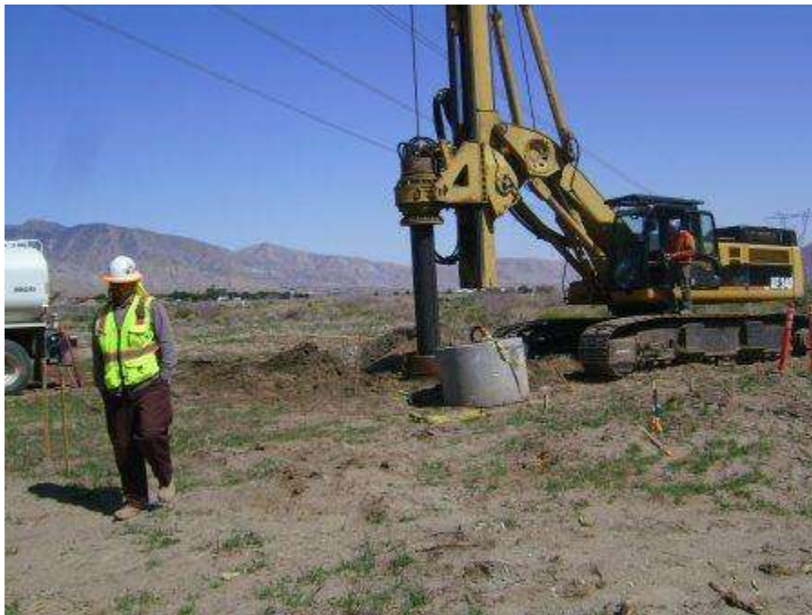
Figure 4. Foundation drilling at Tower 1059
