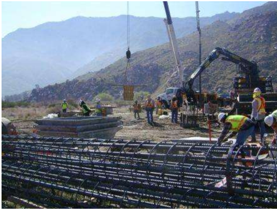
Figure 3. Setting up to pour concrete foundations at Tower 1057.
