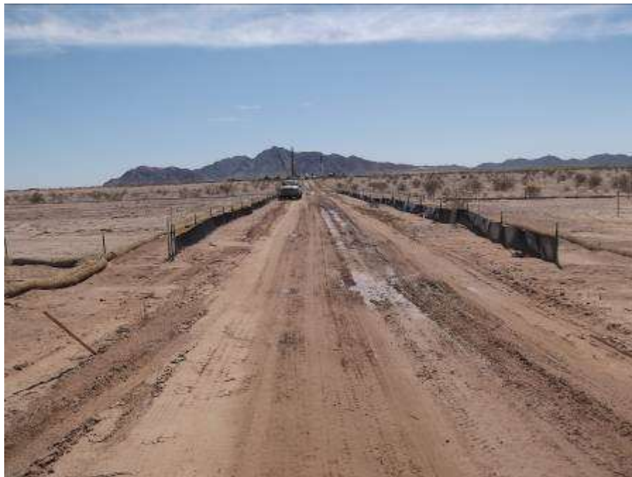
Figure 6. Desert tortoise exclusionary fence modifications along access road between Towers CR1-3W and CR1-4W.
