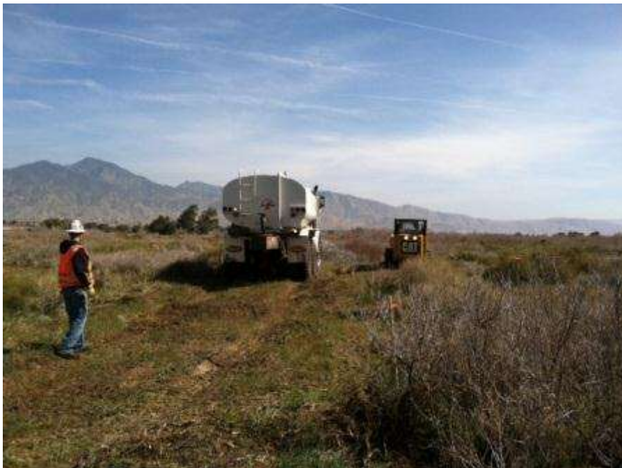
Figure 2. Vegetation clearing on the spur road to Tower 1063/R3.
