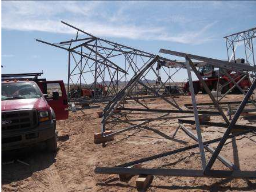
Figure 1. Assembly and erection activities at Towers 2650/CR1-3W.
