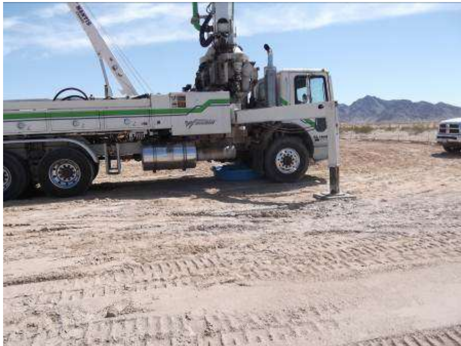
Figure 4. Secondary containment in place during concrete pouring activities at Tower CR1-4W.
