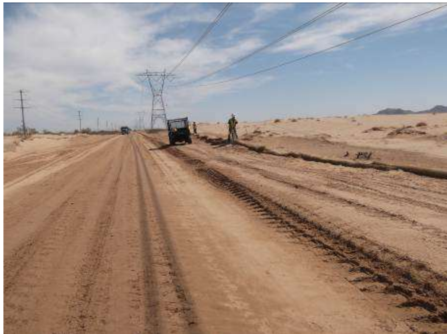
Figure 10. BMP crews maintaining straw wattles along CRS primary access road.
