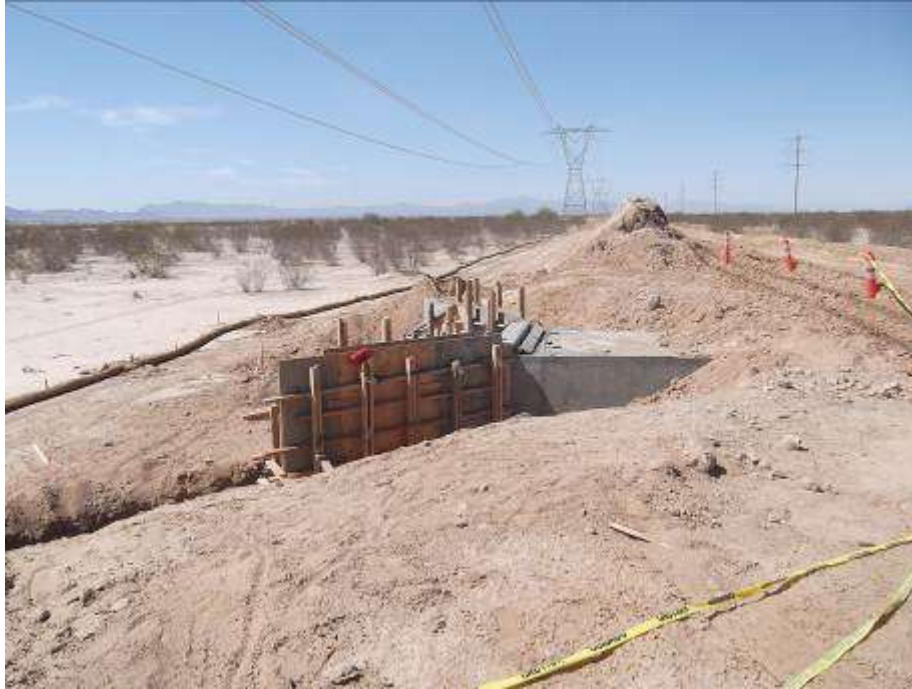
Figure 9. Forms installed for concrete culverts along CRS primary access road.
