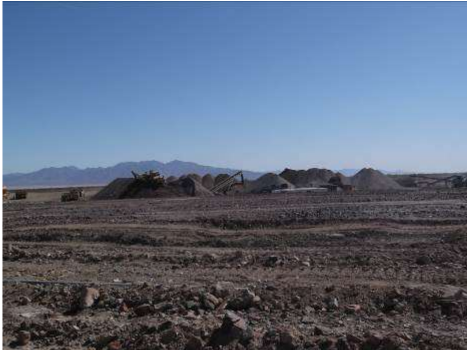
Figure 10. Ongoing rock crushing of native fill at Red Bluff Substation.
