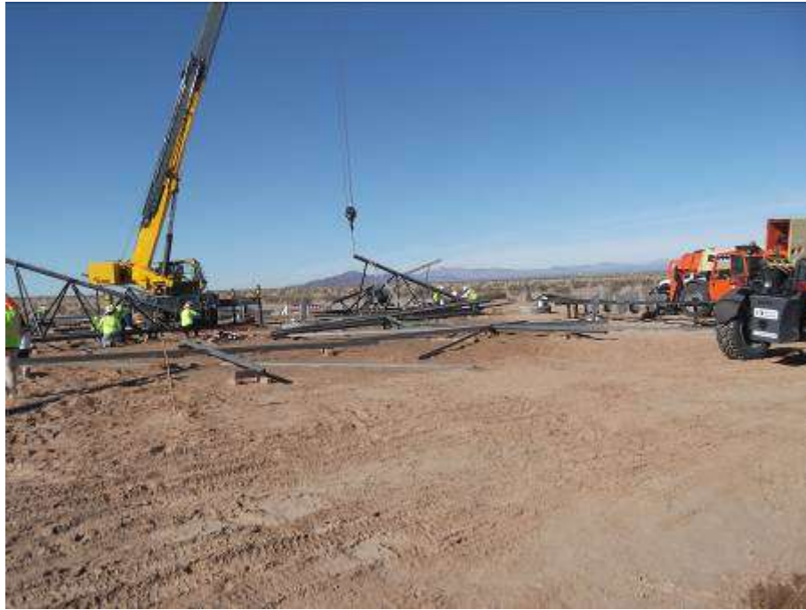
Figure 1. Assembly crews working at Tower CR1-4W.
