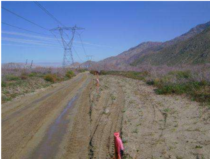
Figure 6. Additional staking was placed in areas where vehicles were driving off of the approved access road between Towers 1061 and 1063.
