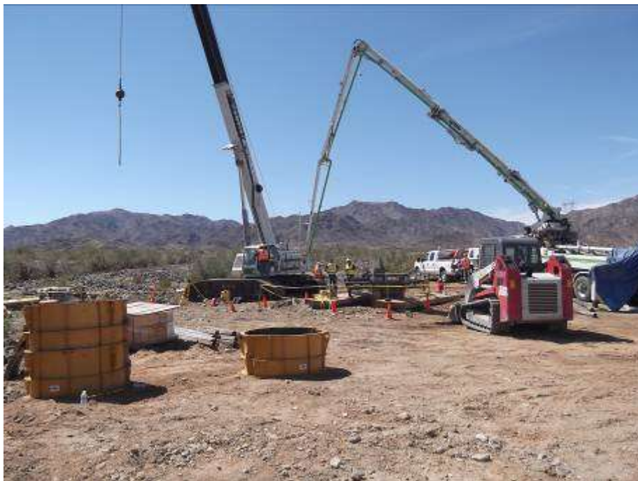
Figure 2. Concrete pouring at Tower RB2-2W.
