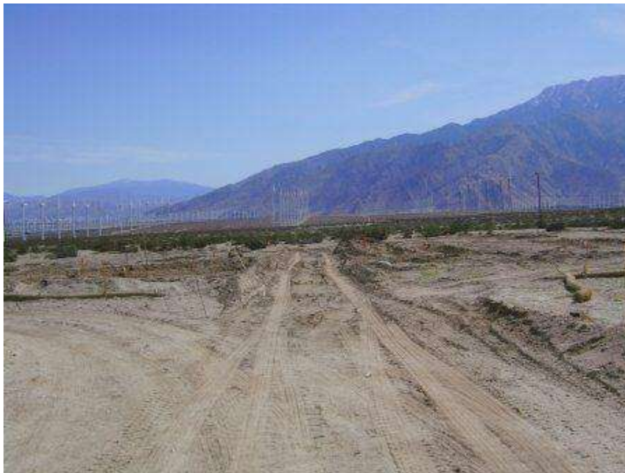
Figure 8. Grading that occurred at Tower 1006 without an archaeological monitor.
