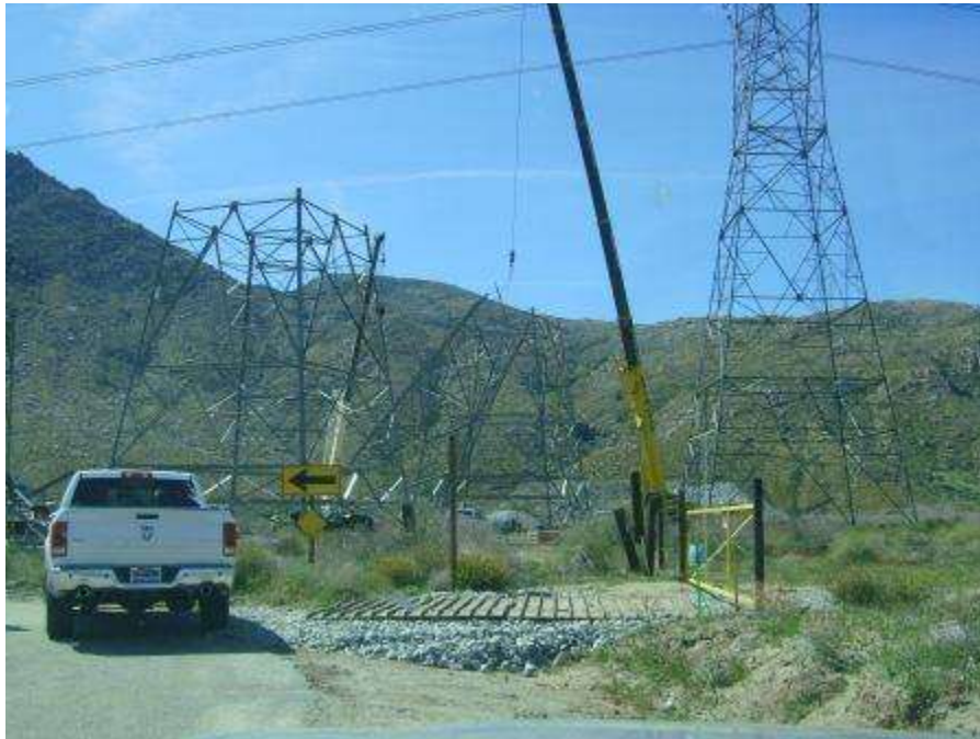
Figure 4. Tower Assembly at Tower 1062 using large crane.
