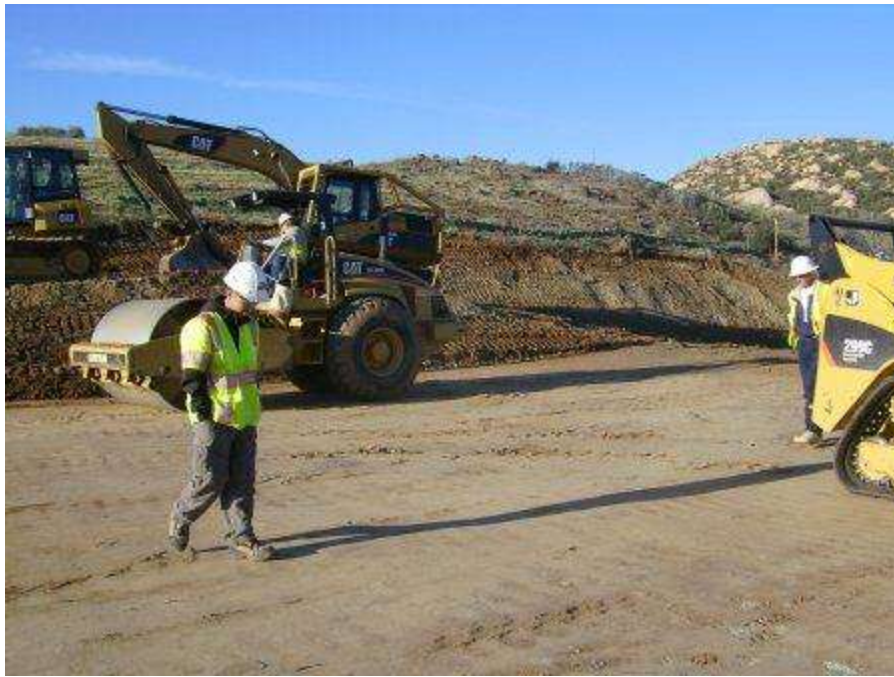
Figure 3. Spur road and crane pad grading at Tower 1091.
