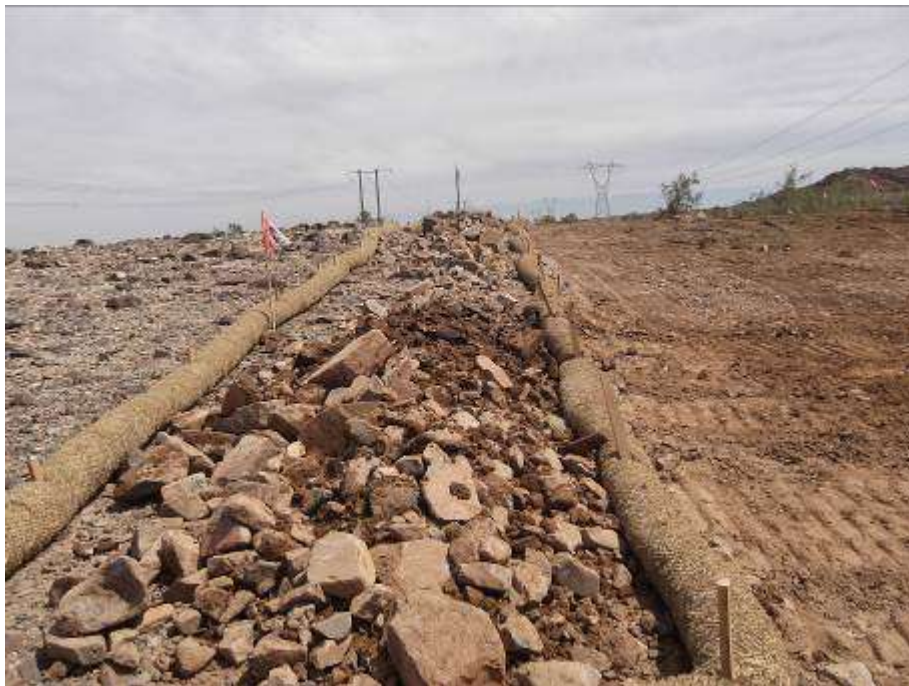
Figure 2. Area defined by BMP boundaries for desert pavement salvage at Tower 2529.
