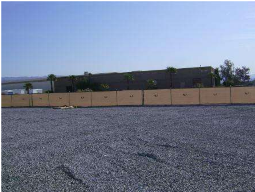
Figure 10. Construction yard screening replaced at Devers 2 Yard.
