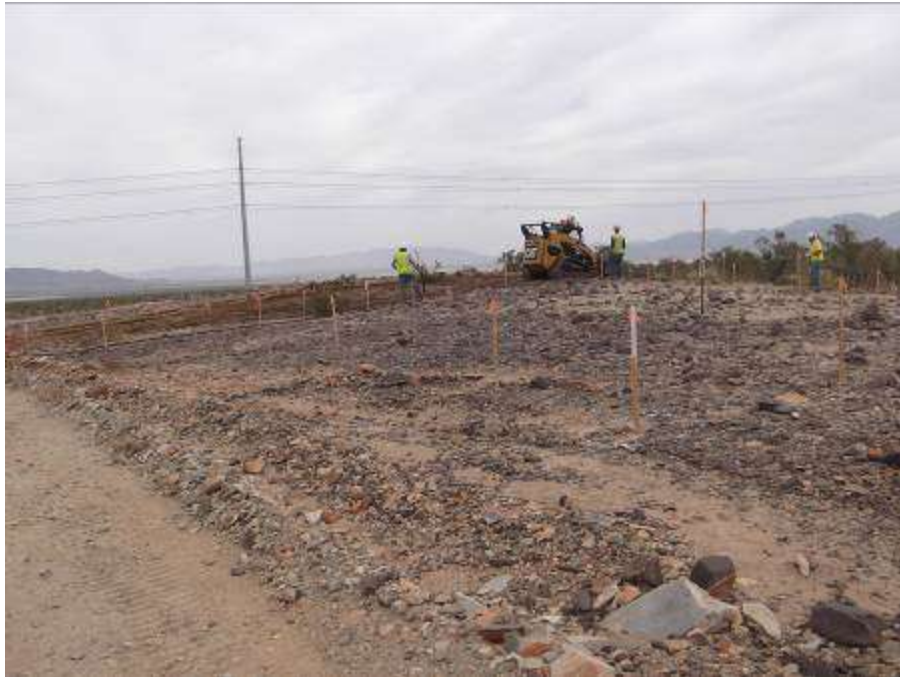
Figure 1. Initiation of desert pavement removal at Tower 2529.
