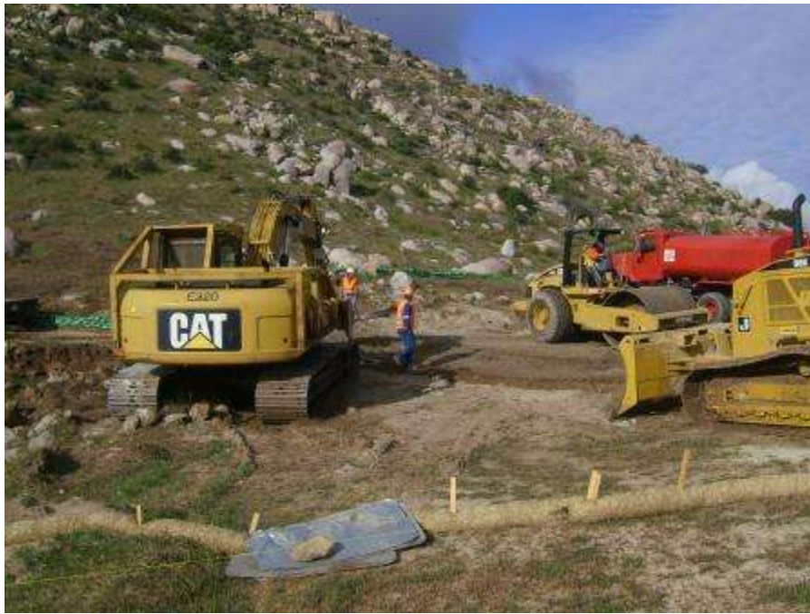
Figure 3. Crane pad grading at Tower 1073.
