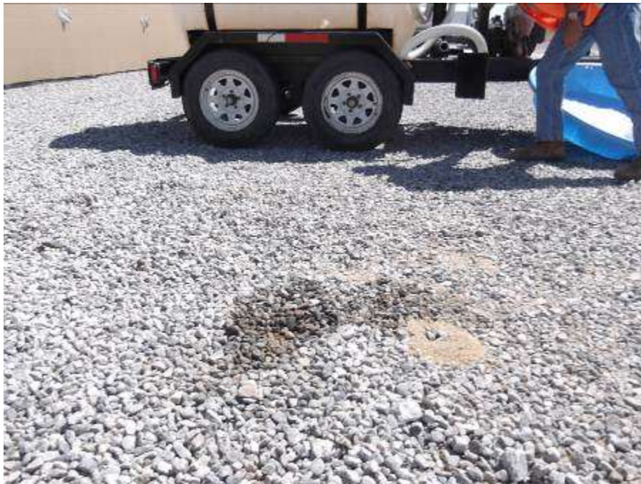
Figure 10. Minor motor oil spill that had not been removed at the Summit Construction Yard.
