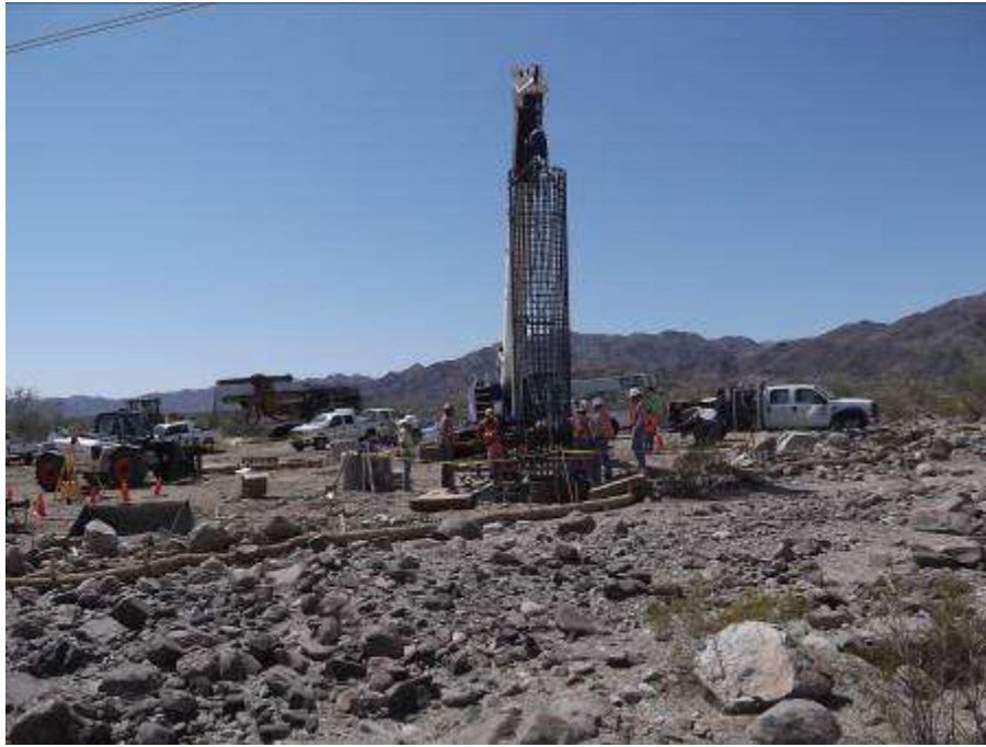
Figure 1. Concrete pouring activities at Tower RB1-5E.
