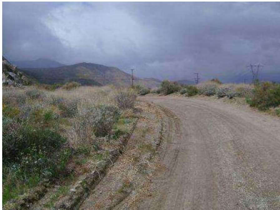
Figure 8. Area on the access road to Tower 1055 where equipment went outside of the access road and crushed vegetation
