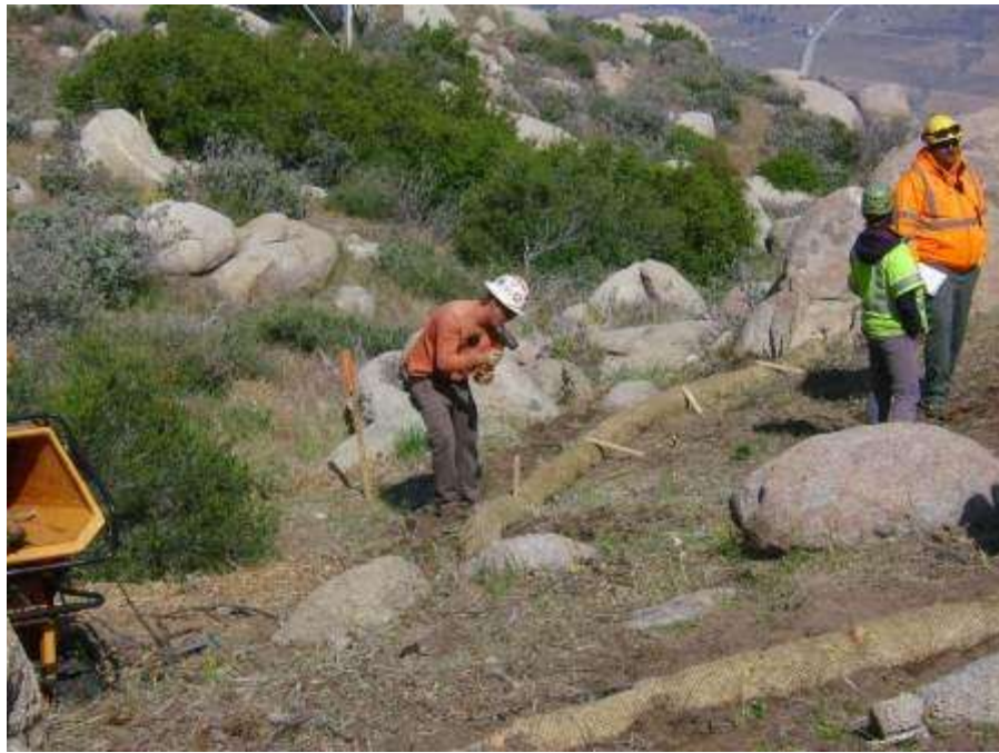
Figure 3. BMP installation at Tower 1047.
