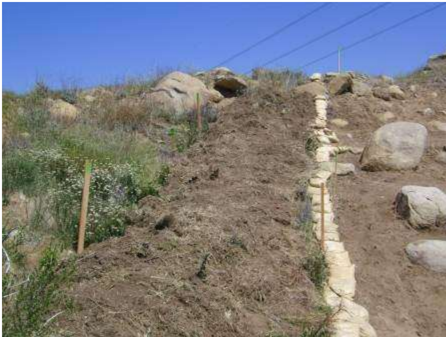
Figure 2. Topsoil salvage at Tower 1071.
