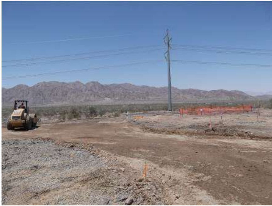
Figure 5. Grading activities occurring while avoiding ESA (right of photo) at Tower 2454.
