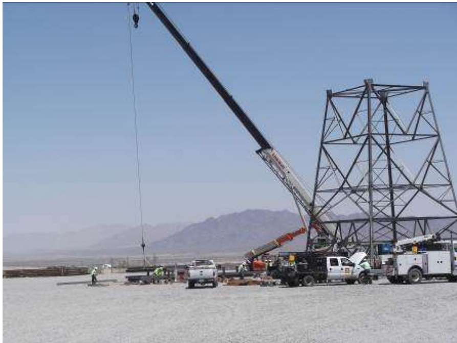
Figure 2. Assembly crew onsite at Tower RB1-3W.
