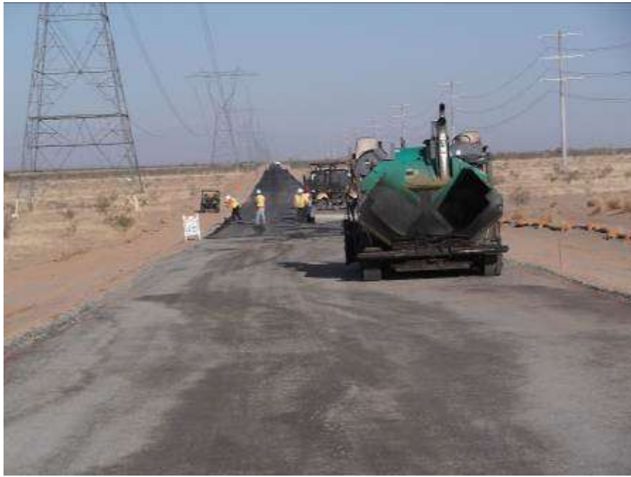
Figure 9. Road paving activities along the primary CRS access road.
