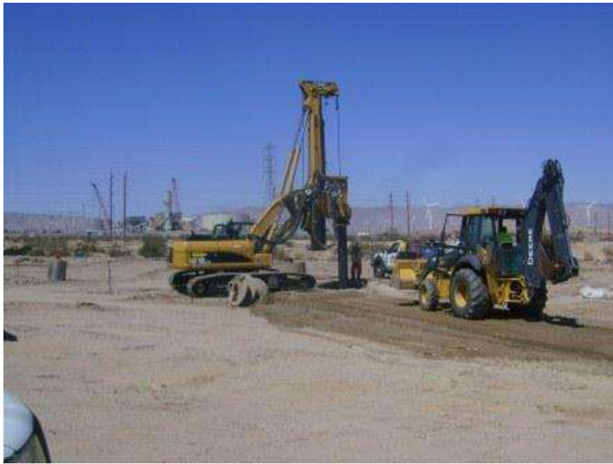
Figure 3. Foundation excavation drilling at Tower 1002.
