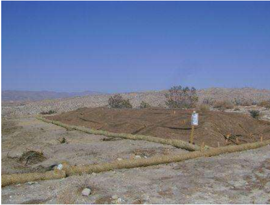
Figure 1. Soil salvage for sensitive plant species at Tower 2107.
