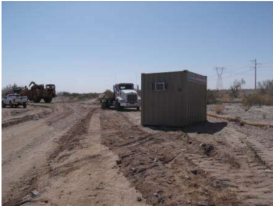
Figure 10. Temporary guard structure installed at intersection of Corn Springs Road and ROW access road.
