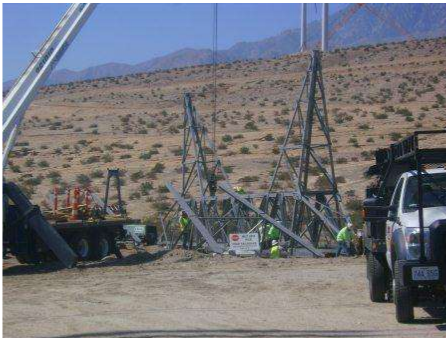
Figure 4. Tower assembly at Tower 1010.
