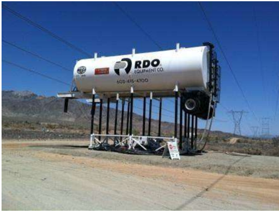
Figure 5. Water Stand Tanks and road base material installed in unapproved area at the ROW entrance near Cactus City Rest Area and Tower 2317.
