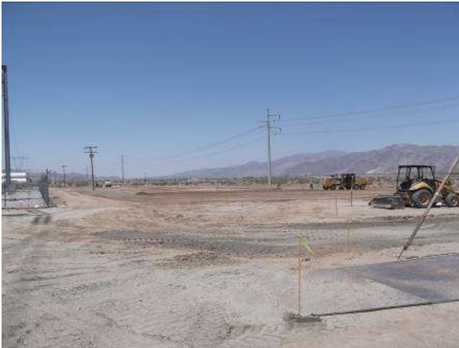
Figure 6. Grading activities conducted at the Series Capacitor expansion site.
