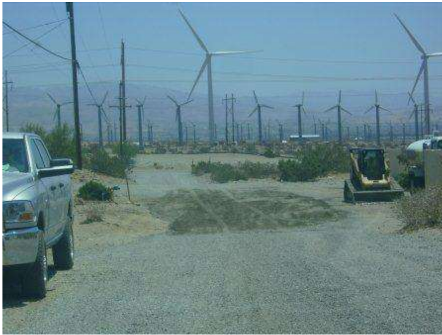
Figure 3. Road maintenance on Smoke Tree Lane at approved water source.
