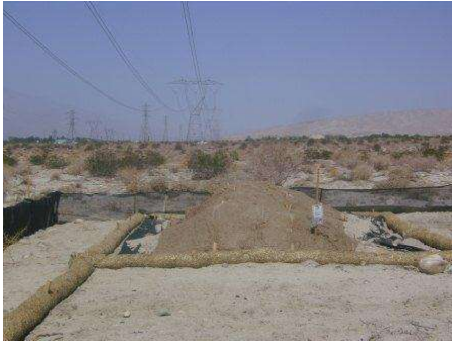
Figure 1. Soil salvage for sensitive plant species at Tower 2133.
