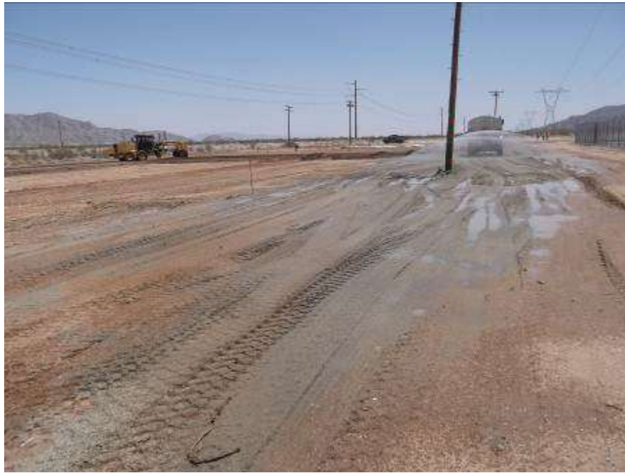
Figure 7. Adequate dust control measures implemented at the Series Capacitor expansion site.
