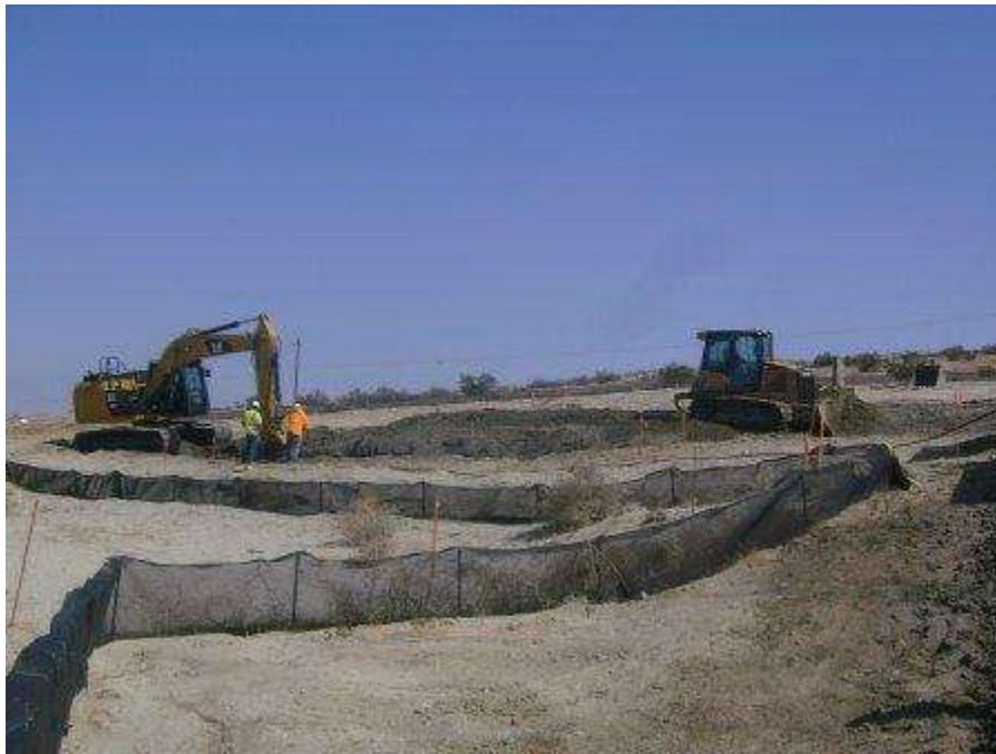
Figure 2. Grading the crane pad for Tower 2113
