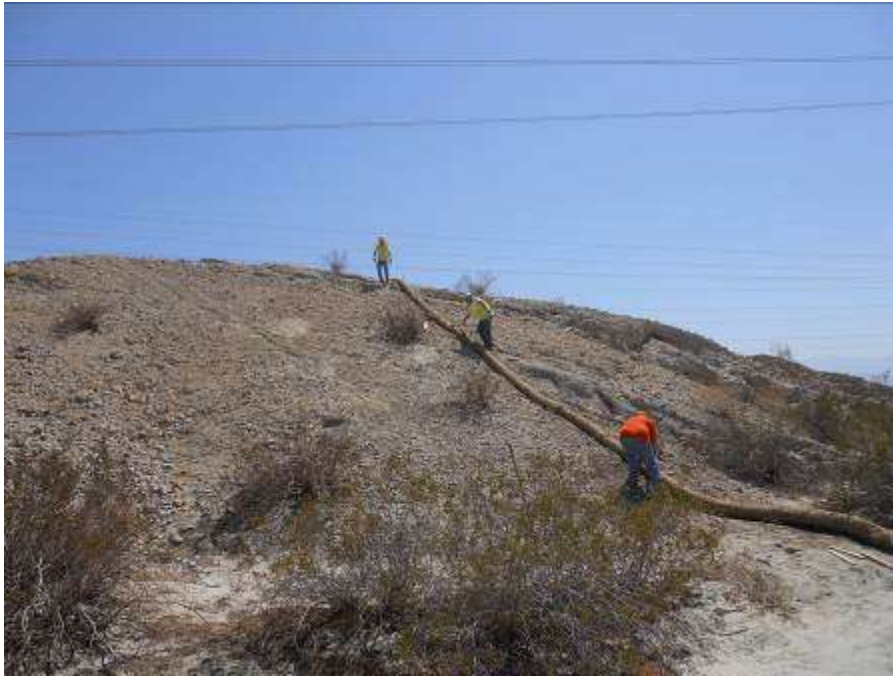
Figure 1. Installation of BMPs at Tower 2232.
