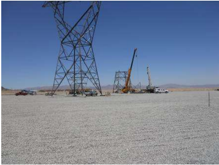
Figure 3. Assembly activities occurring at Tower RB1-4W.
