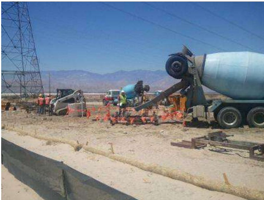
Figure 2. Concrete pouring for foundations at Tower 2127.
