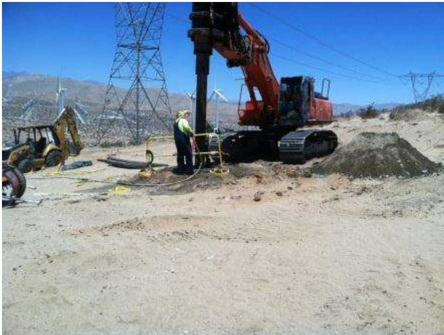
Figure 4. Foundation excavation at Tower 1014.
