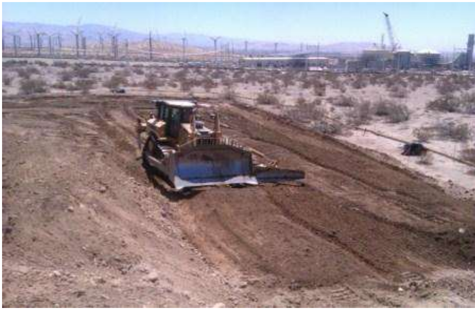
Figure 9. Grading activities within the Expansion Area of the Devers Substation.
