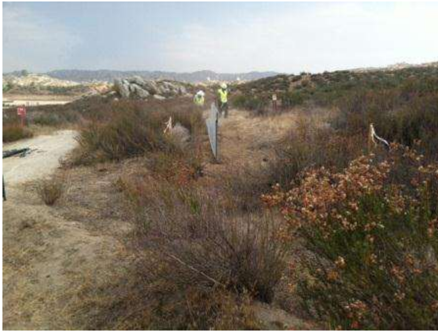
Figure 5. Installation of Stephen's kangaroo rat exclusionary fencing at Tower 1133.
