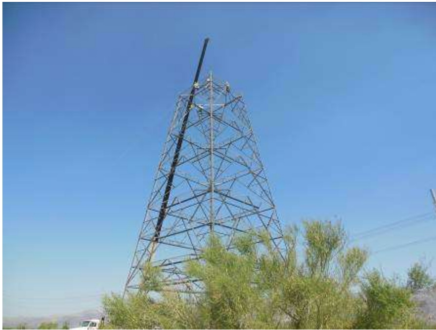
Figure 3. Assembly/erection activities occurring at Tower 2435.
