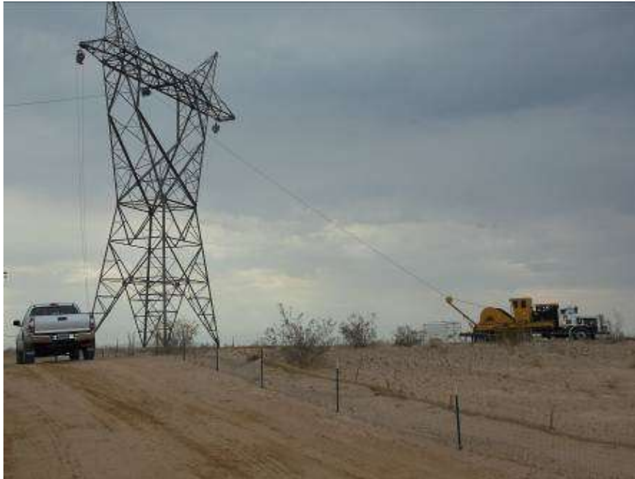
Figure 1. Wire stringing activities occurring at the CRS loop-in tower sites.
