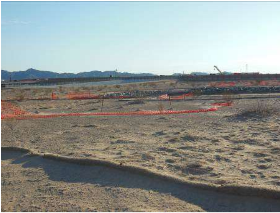
Figure 10. Damaged ESA fencing along the CRS access road.
