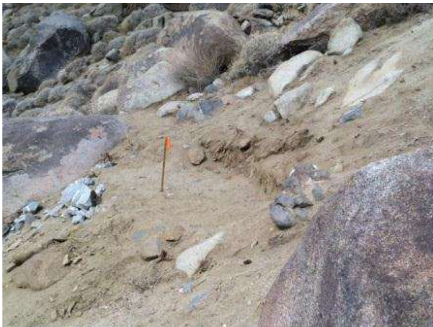
Figure 4. Rock clearing and micropile foundation preparation at Tower 1033.
