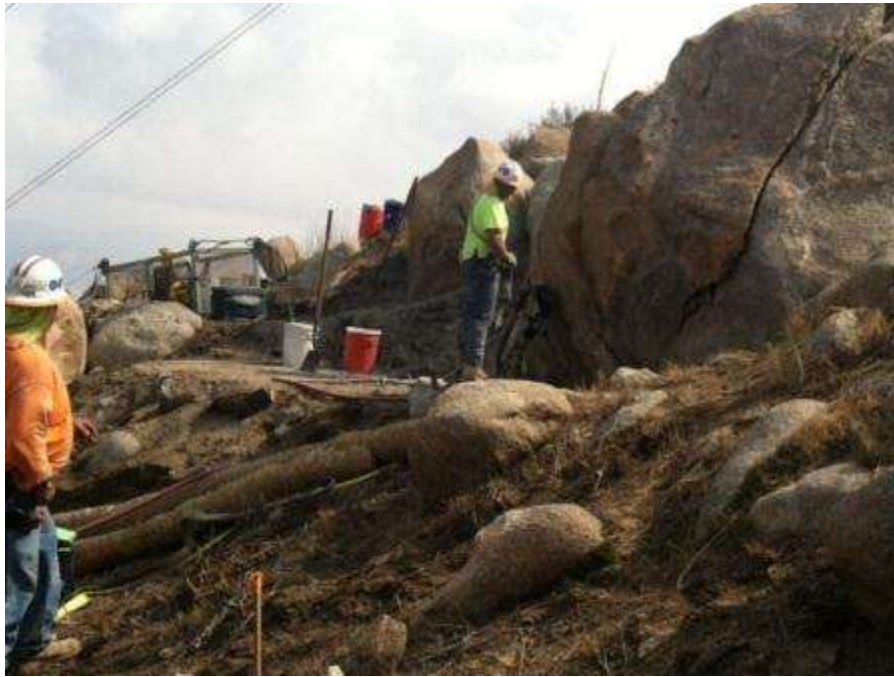
Figure 7. Micropile foundation site preparation at Tower 1049.
