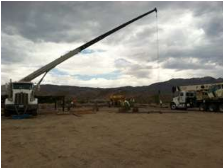
Figure 3. Steel assembly at Tower 2316.
