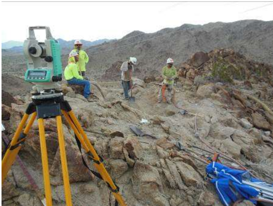
Figure 2. Excavation of micropile foundations at Tower 2424.
