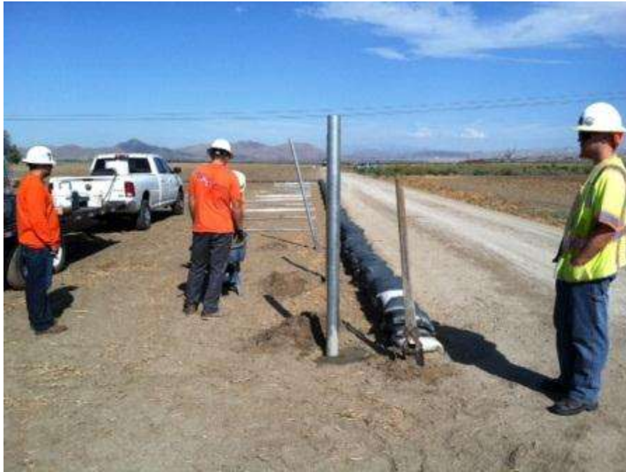
Figure 5. Installation of perimeter fencing at HLZ H9.
