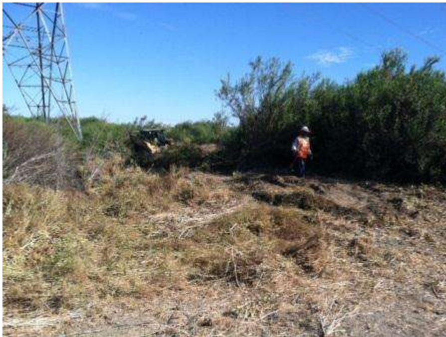
Figure 6. Site vegetation clearing at Tower 1120.
