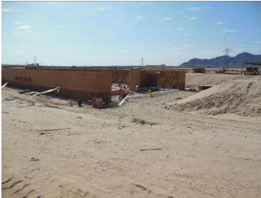
Figure 9. Construction of the MEER building at CRS.
