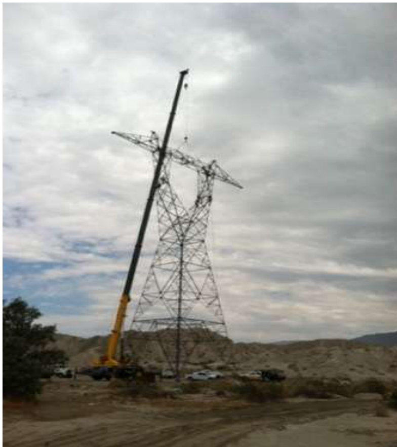
Figure 4. Steel erection at Tower 2239.
