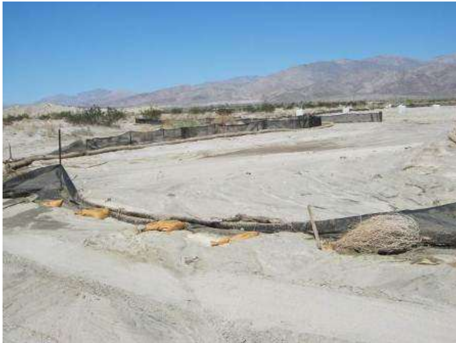
Figure 6. Coachella Valley Fringe-toed lizard fencing and BMPs damaged by a storm at Tower 2341.
