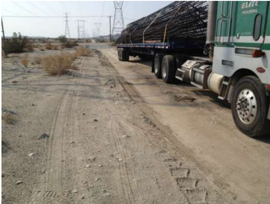
Figure 5. Tire tracks in sandy soil resulting from a project vehicle driving seven feet outside of the access road limits for 130 feet near Tower 2242.
