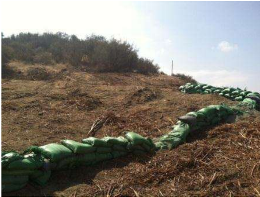
Figure 7. Tracks left outside the disturbance area of Tower 1137 when a dozer was stolen and driven cross country. The gravel bags in the forefront of the photo were also damaged when driven over.
