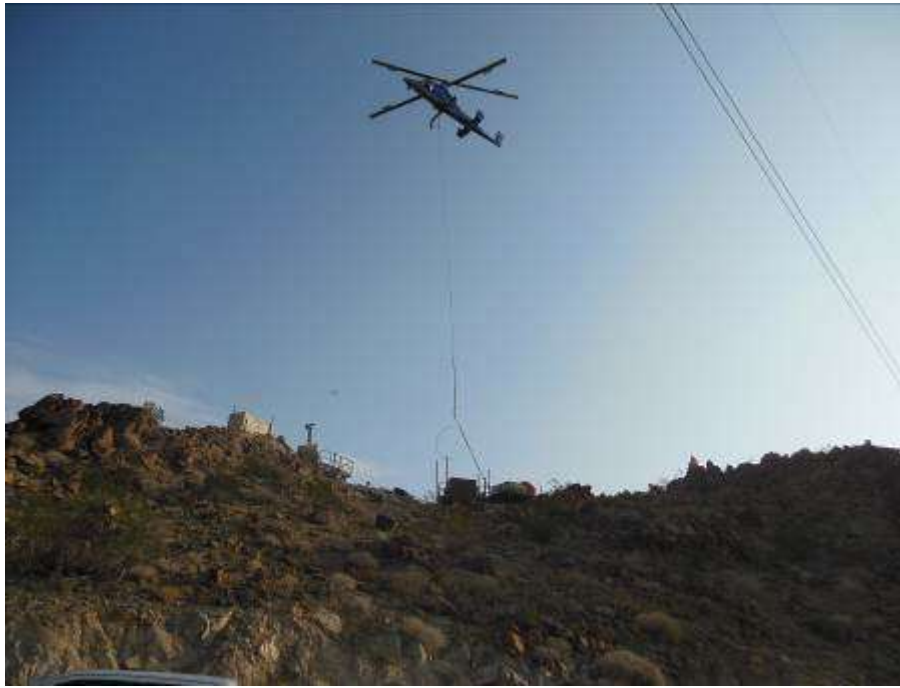
Figure 3. Helicopter transporting materials during micropile drilling activities at Tower 2424.
