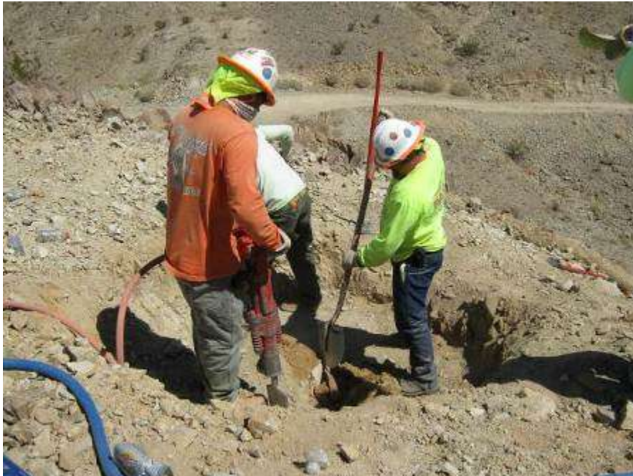
Figure 2. Micropile foundation site preparation at Tower 2310.
