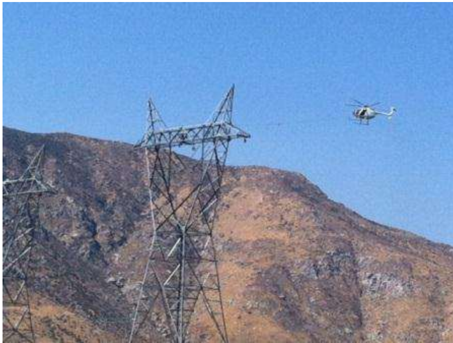
Figure 4. Wire stringing activities at Tower 1062. The helicopter is pulling the sockline.
