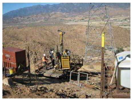
Figure 5. Micropile foundation drilling at Tower 1068.
