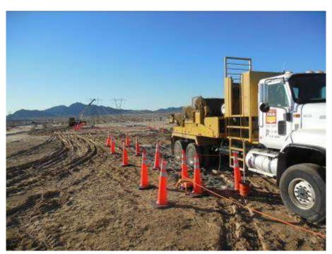
Figure 2. Stringing activities associated with the western CRS loop-in towers.
