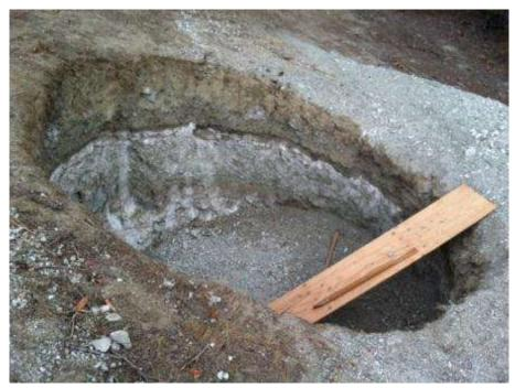
Figure 7. Wildlife ramp in place at Tower 1107 to prevent wildlife entrapment.
