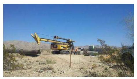
Figure 3. Foundation drilling at Tower 2265.
