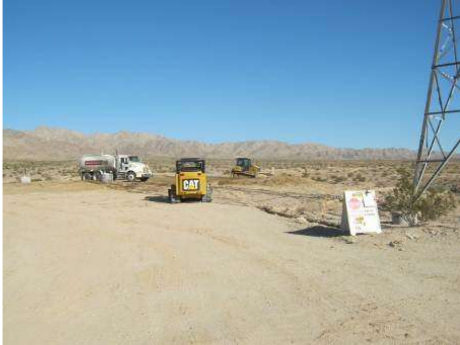
Figure 1. Grading at Tower 2258.
