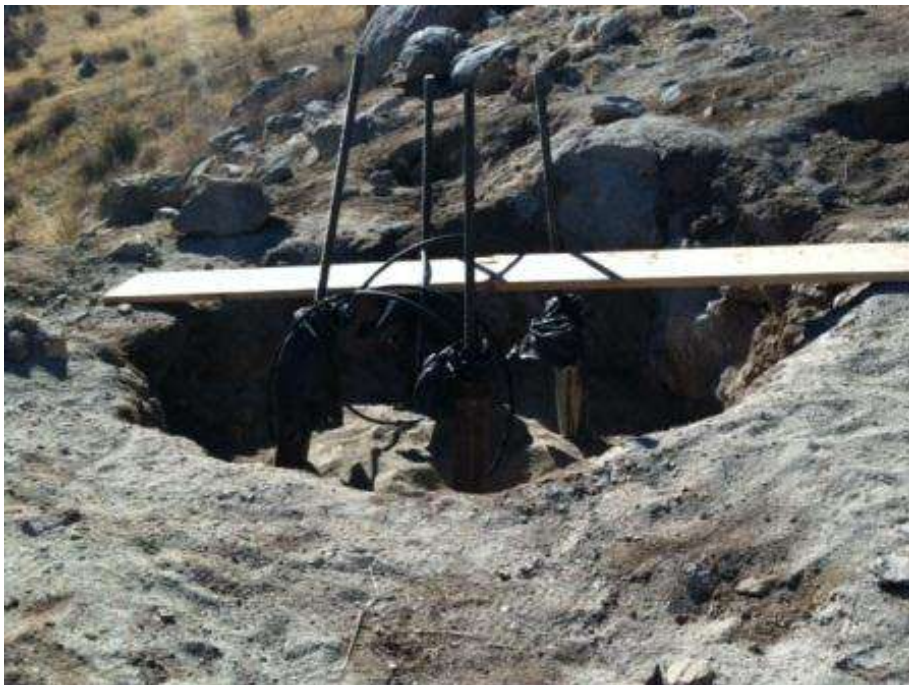
Figure 6. Ineffective wildlife ramp at Tower 1067.
