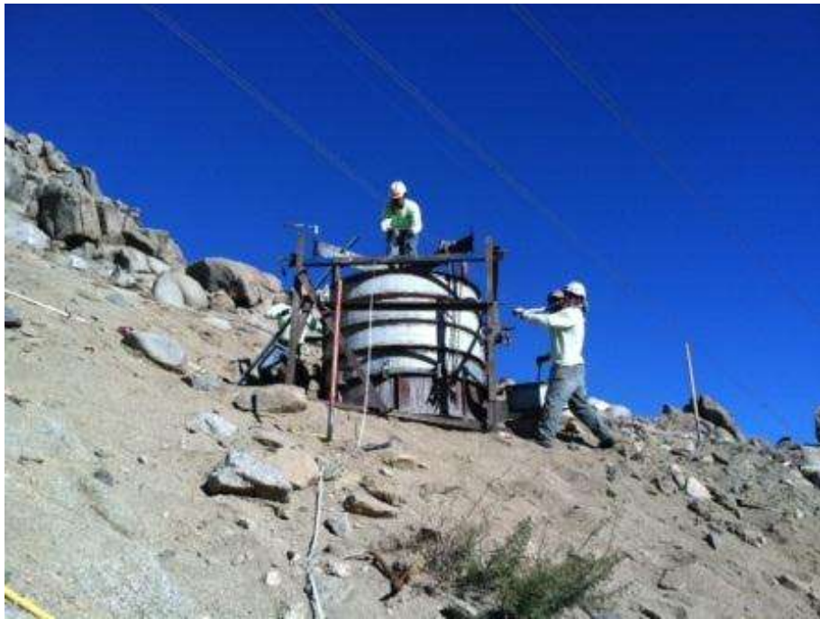
Figure 4. Micropile foundation pile cap preparation at Tower 1033.
