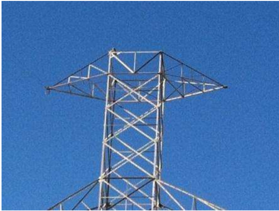
Figure 3. Installation of FAA Lighting on Tower 2000X.
