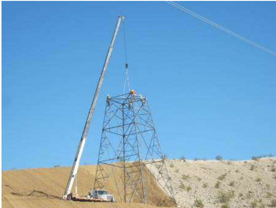
Figure 2. Assembly at Tower 2244.
