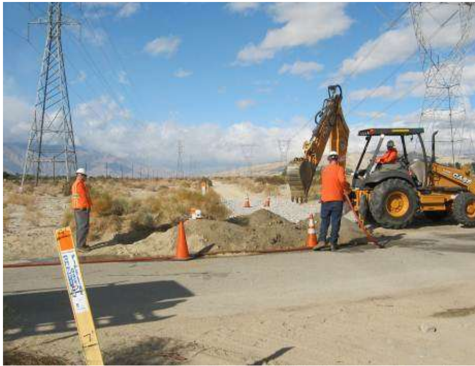
Figure 3. Trenching activities associated with the Mirage Substation Loop-Ins.
