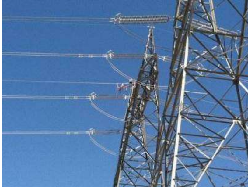
Figure 1. OPGW repair work at Tower 2015.
