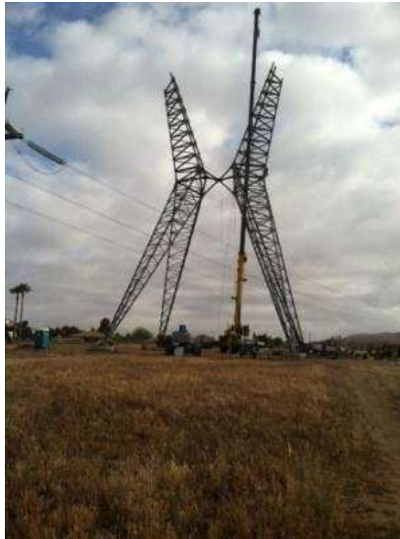
Figure 3. Tower assembly at Tower 1153.
