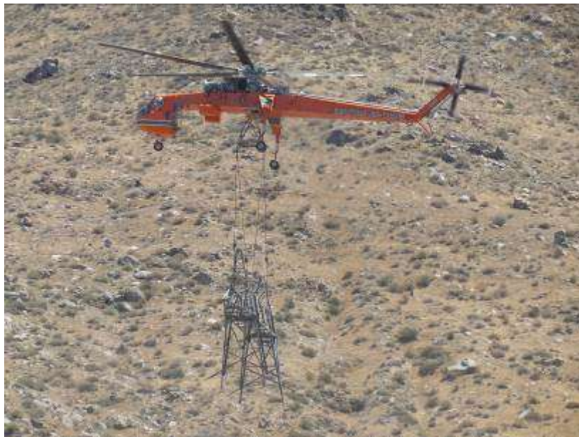
Figure 4. Hauling tower bridge from HLZ H2.
