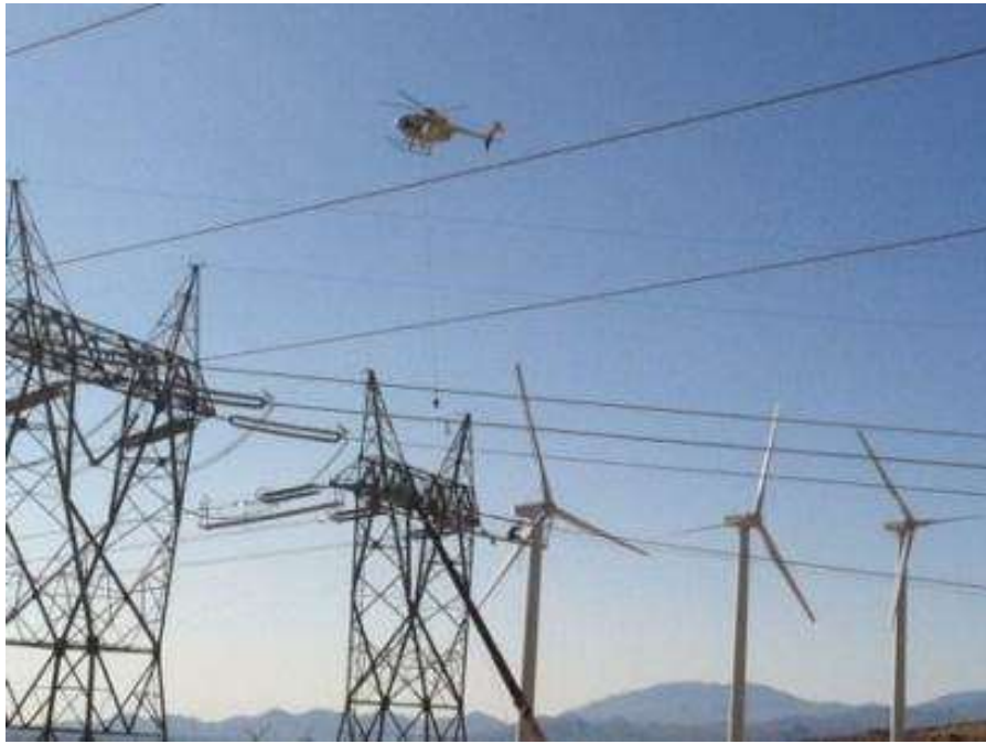
Figure 5. Wire stringing activities at Tower 1010.
