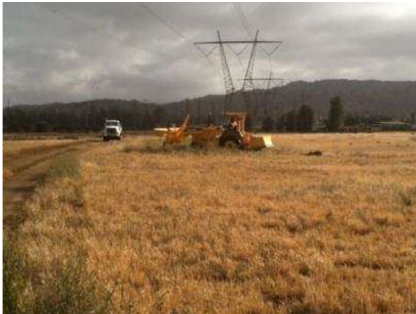
Figure 2. Site clearing at Wire Site 49.
