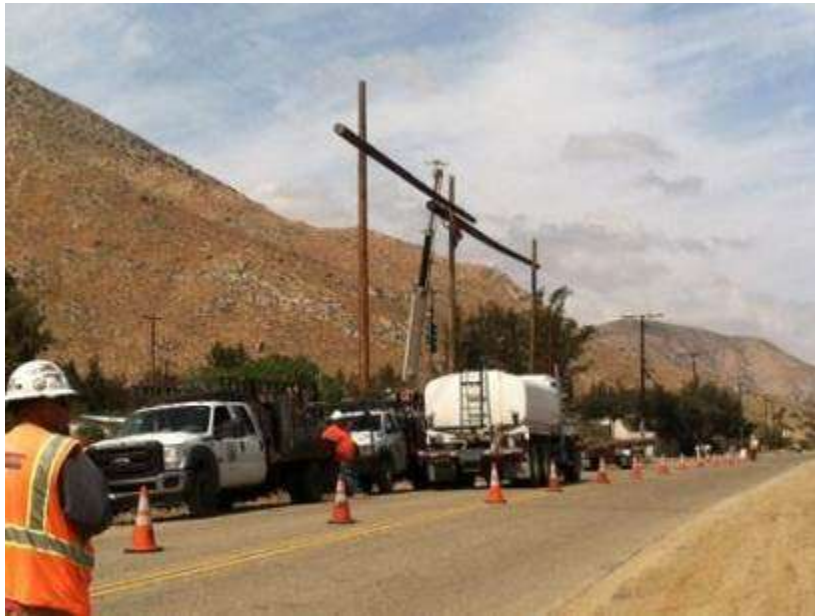
Figure 3. Guard pole installation on Esperanza Ave. near Tower 1054
