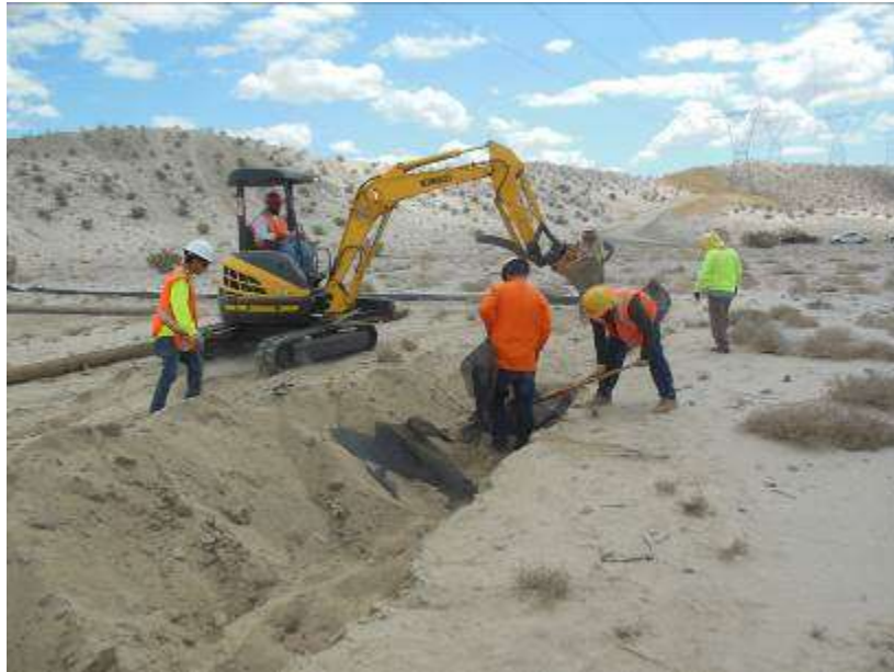
Figure 1. Removal of CVFTL exclusionary fencing at Tower 2243.
