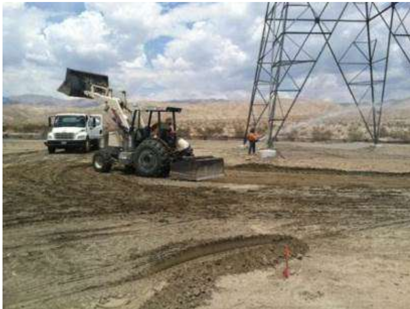
Figure 2. Site stabilization activities at Tower 2211
