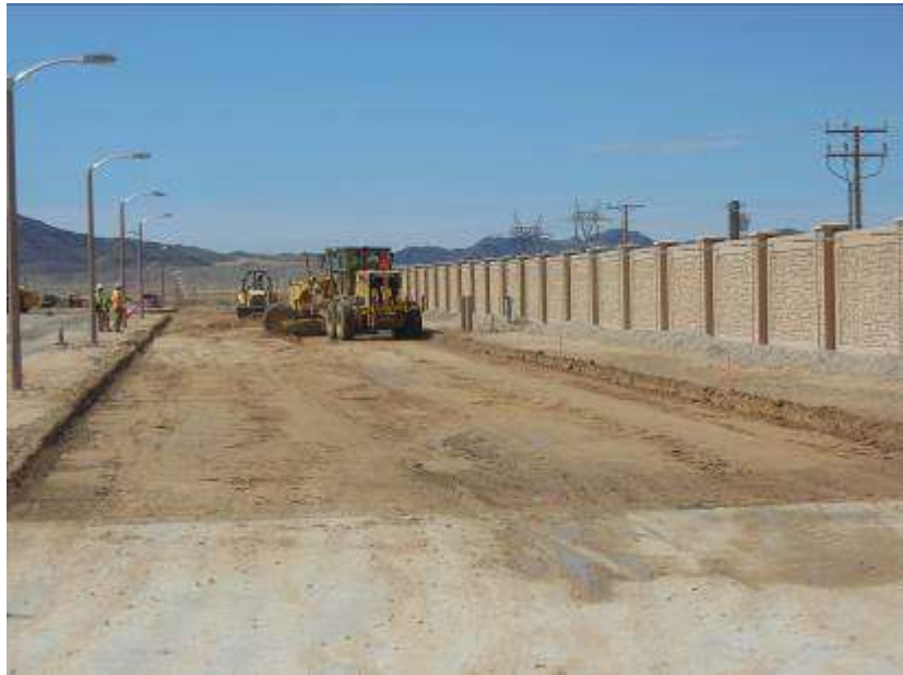
Figure 7. Fine grading of access road within the CRS limits.
