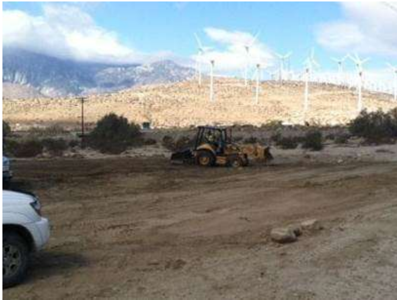
Figure 5. Site stabilization activities at Tower 1007
