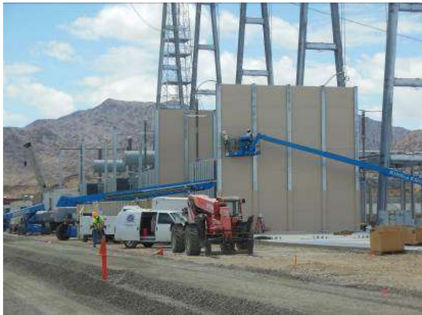
Figure 8. Installation of transformer panels at Red Bluff.
