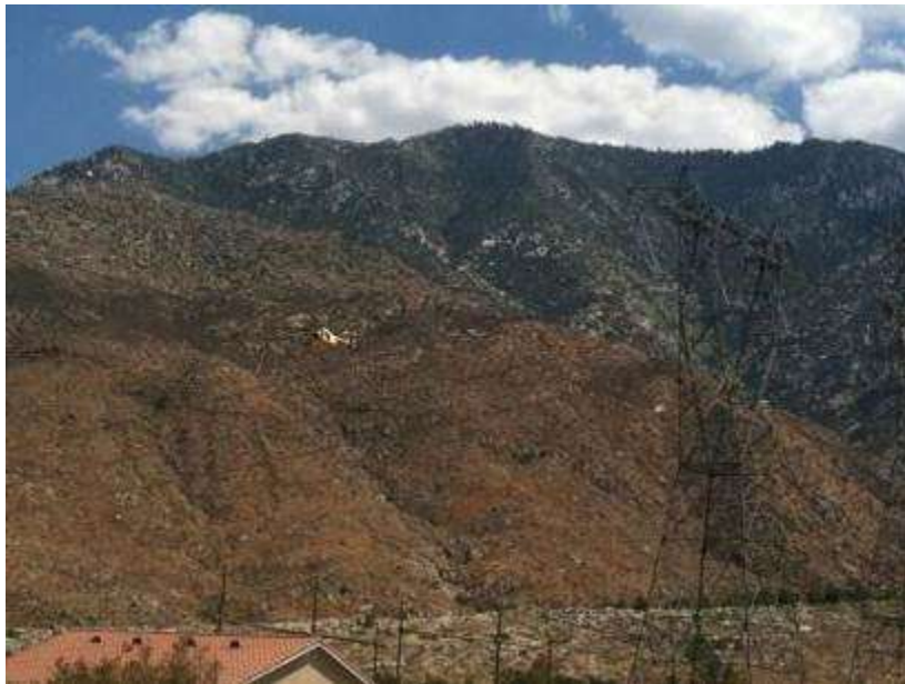
Figure 5. Helicopter wire pulling activities near Tower 1053
