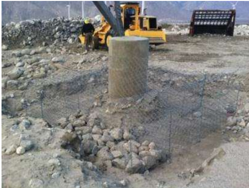
Figure 2. Gabion basket installation at Towers 1017.
