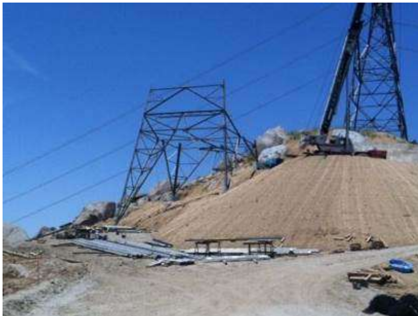
Figure 4. Tower assembly at Tower 1127
