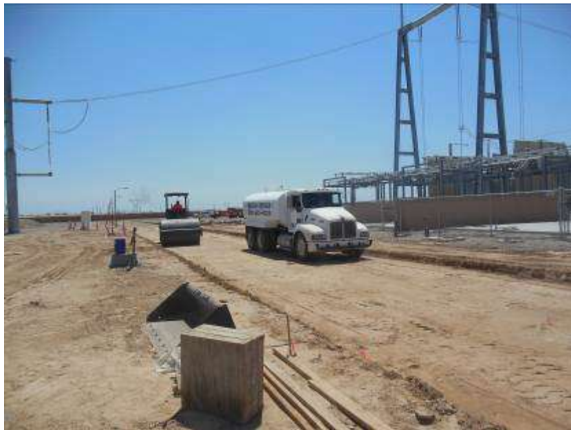
Figure 8. Interior road preparation work at CRS.
