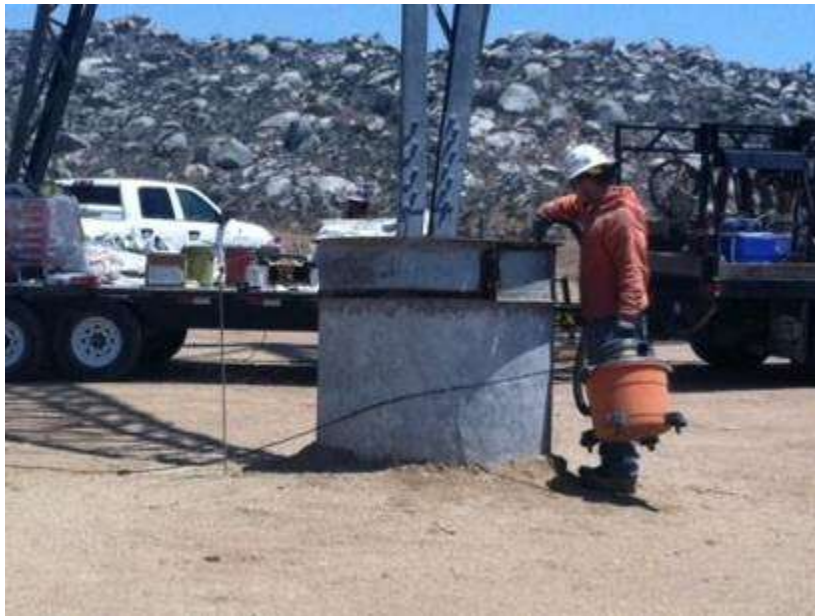
Figure 3. Tetra Tower pilecap finishing at Tower 1146
