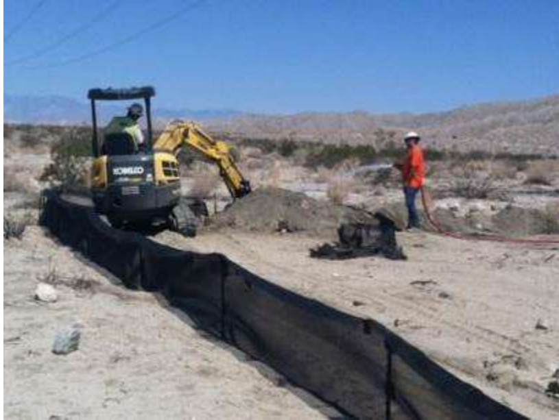
Figure 1. CVFTL fencing removal at Tower 2207
