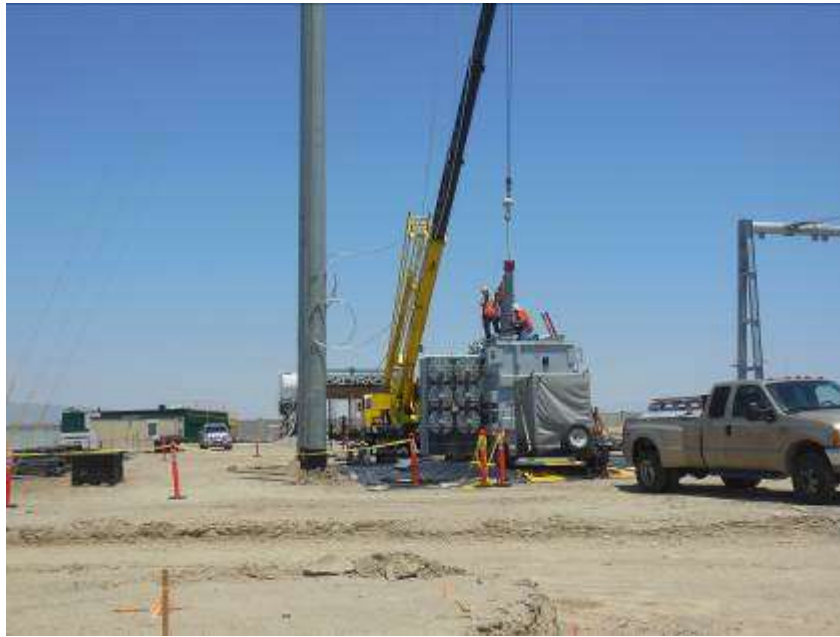
Figure 9. Installation of electrical equipment at Red Bluff.
