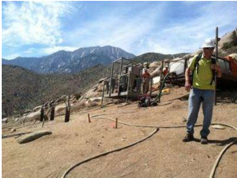
Figure 4. Permanent platform grouting operations at Tower 1037.
