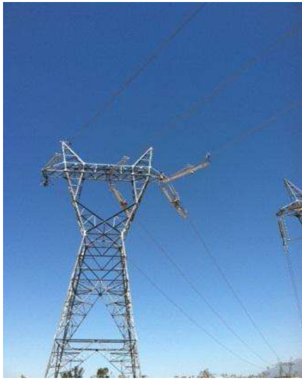
Figure 3. Wire stringing activities at Tower 1054.
