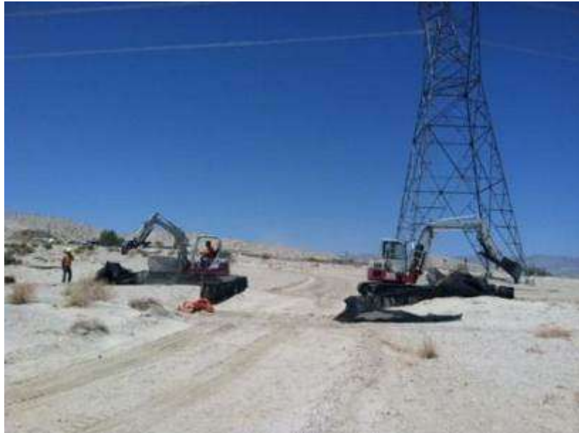
Figure 1. CVFTL fencing removal at Tower 2122.
