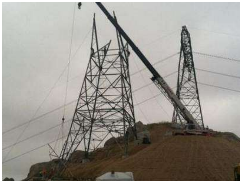
Figure 2. Tower assembly at Tower 1127.
