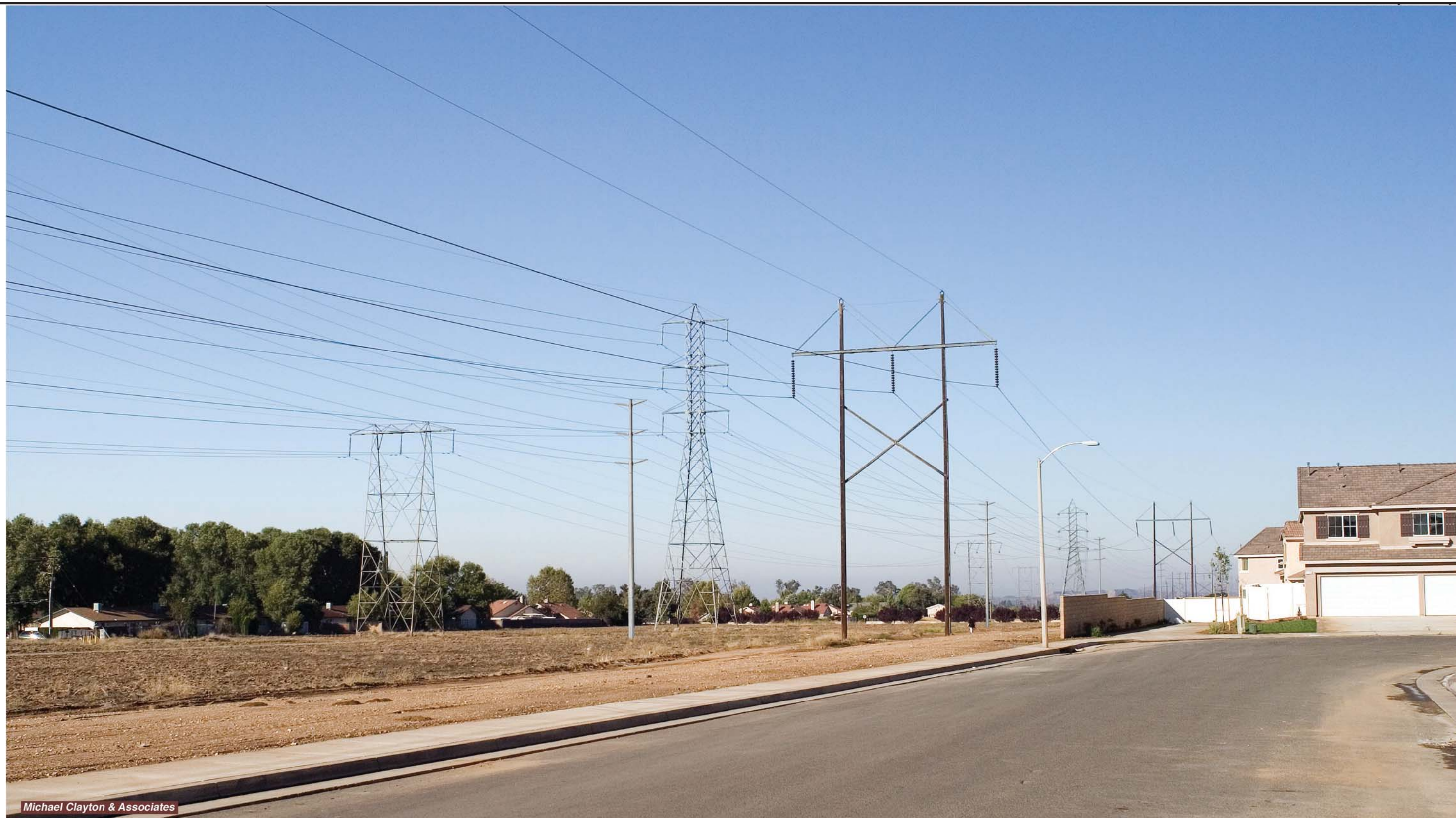
A visual simulation of Route Alternative Option 3 from Key Viewpoint 12 on Cedar Hollow Road approximately mid-block, which is located immediately south of Beaumont High School in the City of Beaumont. This simulation illustrates the introduction of the new 115 kV steel pole subtransmission line between the Devers-Vista Nos. 1 and 2 220 kV transmission lines on the tall lattice steel structures and the Devers-San Bernardino #2 220 kV transmission line on the wood pole H-frame structures to the north (right).
