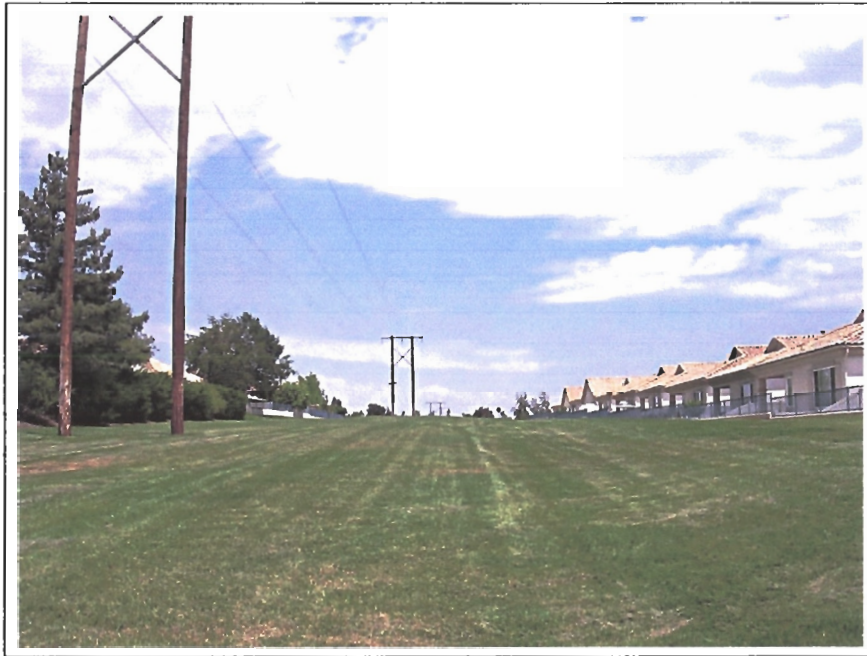
Existing view of 115 kV subtransmission line from Key Viewpoint #5.
