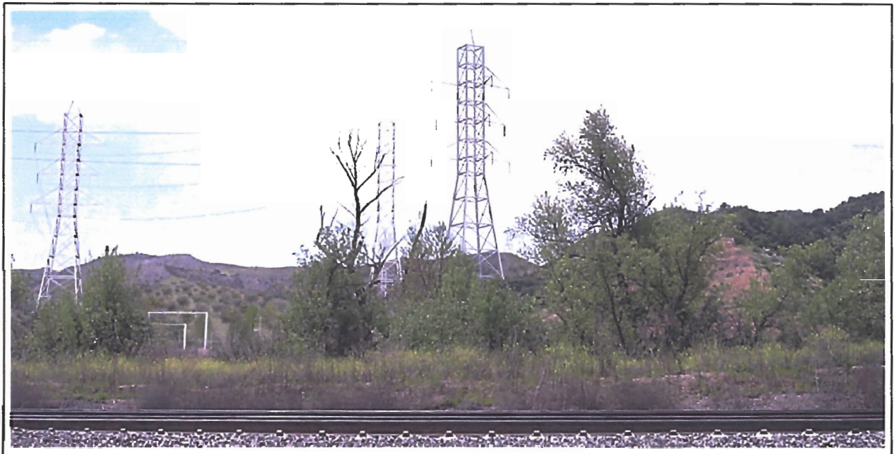
Simulated view of El Casco Substation Site from Key Viewpoint #3.
