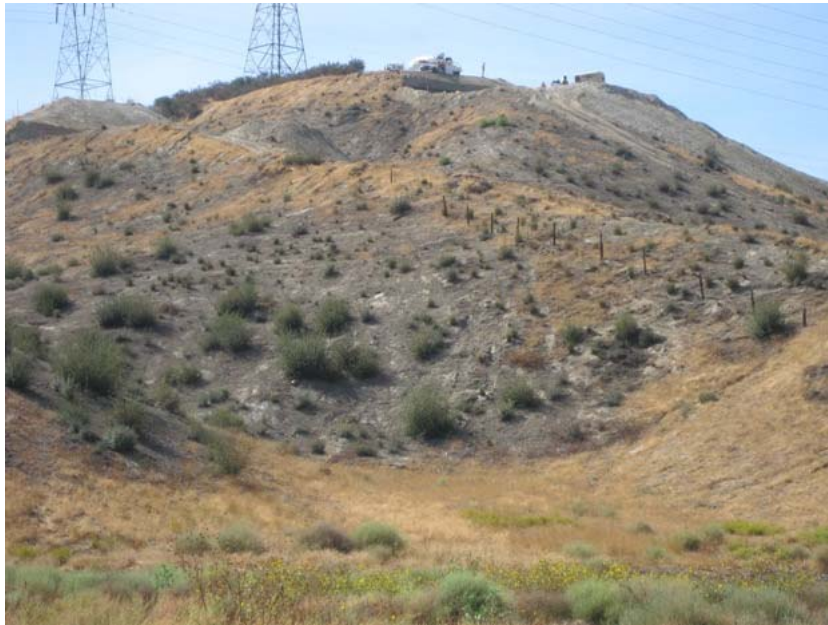
Figure 6: Geologists have determined there is a layer of clay within the hill that has approximately the same slope as the hillside. Building of the substation will require the removal of the toe of the slope. This removal may increase the likelihood of slippage of the material above the clay layer. The intended function of the tension cable anchor system is to put pressure on the clay layer and thereby prevent land slippage. The photograph faces southeastward.
