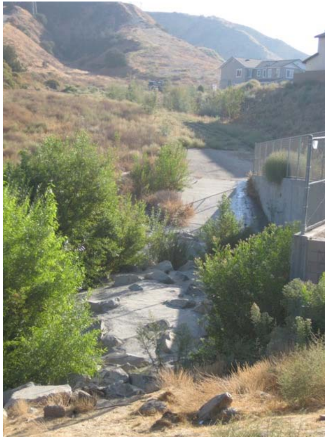
Figure 2: The water source for the auxiliary elevated water tower will be a hydrant at the end of a cul-de-sac in Fairway Estates housing development (in the background). The four-inch above-ground pipeline will cross a small creek and riparian area on the concrete skirting in the foreground. The pipe will connect to the water tower that will be situated at the edge of San Timoteo Canyon Road.
