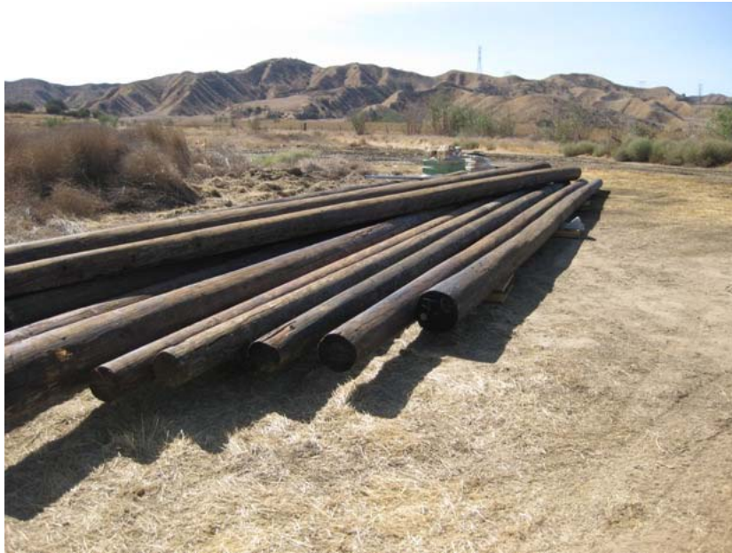
Figure 7: Poles for installation of a utility line from San Timoteo Canyon Road to the El Casco Substation site were brought to the site during the subject week. They have been stored on pallets to prevent creosote contact with the soil. The photograph was taken just inside the entrance gate and faces westward.
