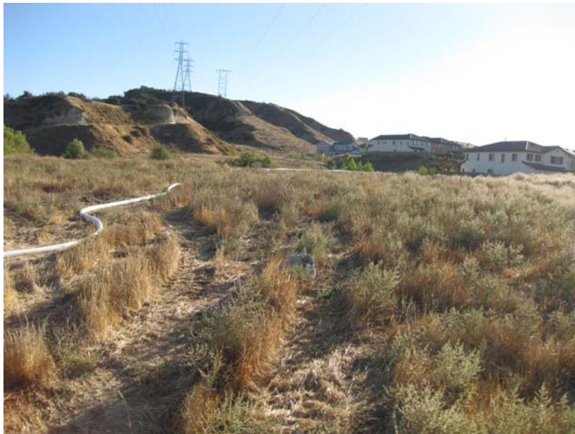
Figure 4: The water for the second water pipeline/tower system for the El Casco Substation construction is piped from a hydrant in an adjacent housing development in the distance. The water tower is behind the photograph, which faces northeastward.
