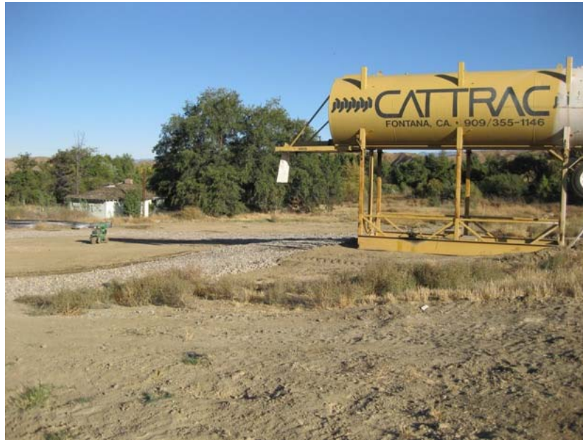
Figure 5: The second water tower is adjacent to San Timoteo Road (to the left of the photograph). The tower area has been fitted with a shaker plate, a gravel loop road for water loading, a perimeter fence and gate, and a silt fence for run off prevention. The photograph faces westward.
