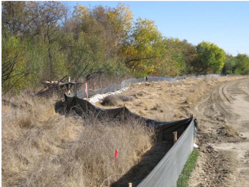
Figure 2: During the subject period, the silt fence previously located at the northern edge of the pre-existing access road was moved closer to the San Timoteo Creek bank adjacent to the substation site. Note the sand bags at the base of the fencing for additional water runoff containment. The photograph faces eastward.
