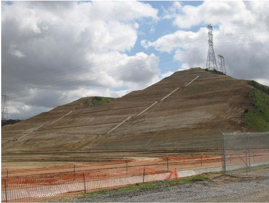
Figure 1: View of completed terraced slope at El Casco Substation. Note the newly installed V-ditches. The photograph faces southeast.
