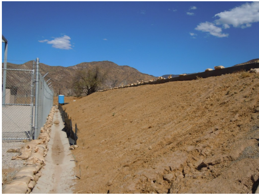
Figure 3: At the Zanja Substation site no germination was evident at one of the hydroseeded areas. The photo is taken facing north.
