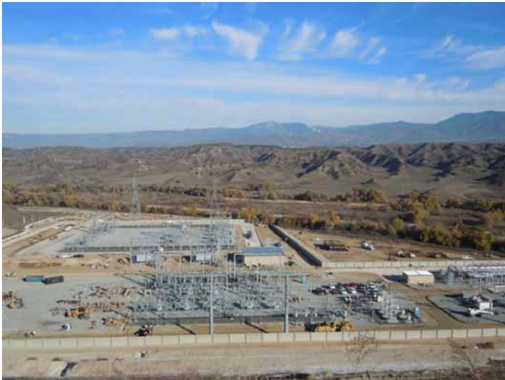
Figure 4: At the El Casco Substation site, a panoramic view of the substation.
