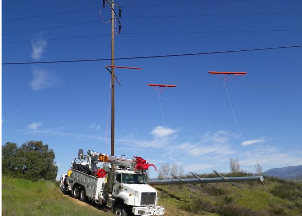
Figure 1: View of crews installing pole 213 on Segment 7. The photograph faces northwest.
