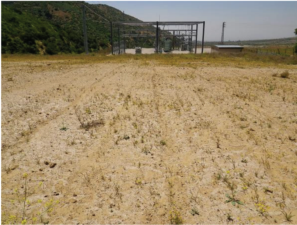
Figure 3: View of hydroseeded temporary work area at Zanja Substation. The photograph faces west.
