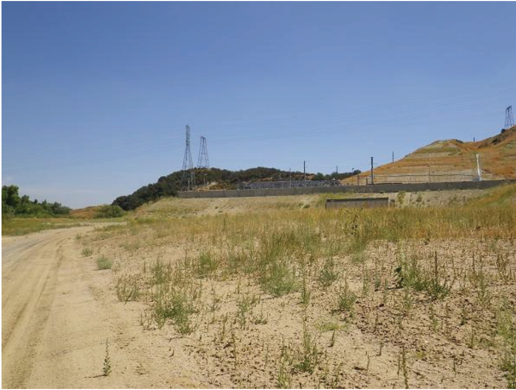
Figure 1: View of hydroseeded temporary work areas near the El Casco Substation. The photograph faces east.
