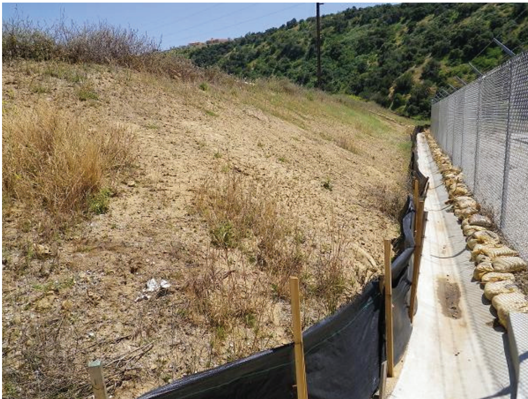
Figure 4: View of hydroseeded temporary work area at Zanja Substation. The photograph faces south.
