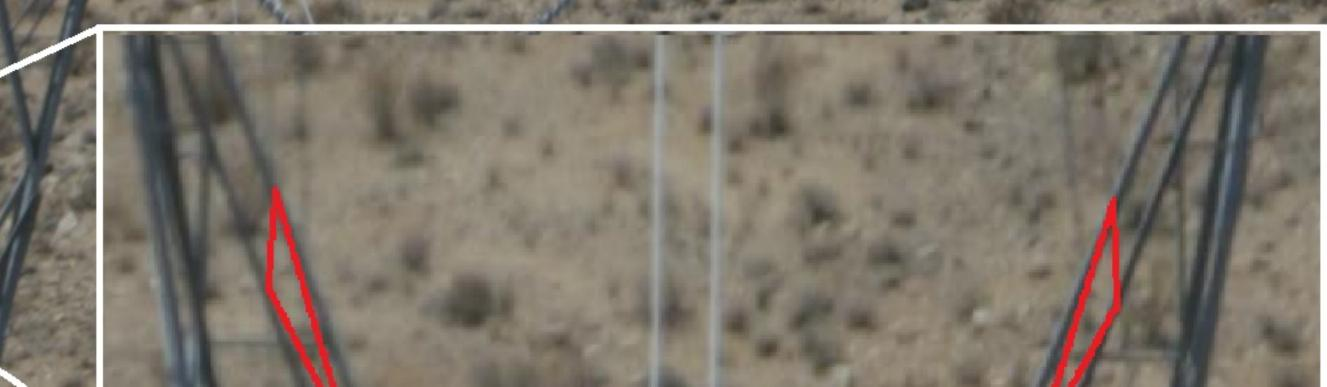
BODY MODIFICATIONS: X-BRACES ADDED TO "LAYBACKS" TO SUPPORT OPGW SPLICE LOCATION
