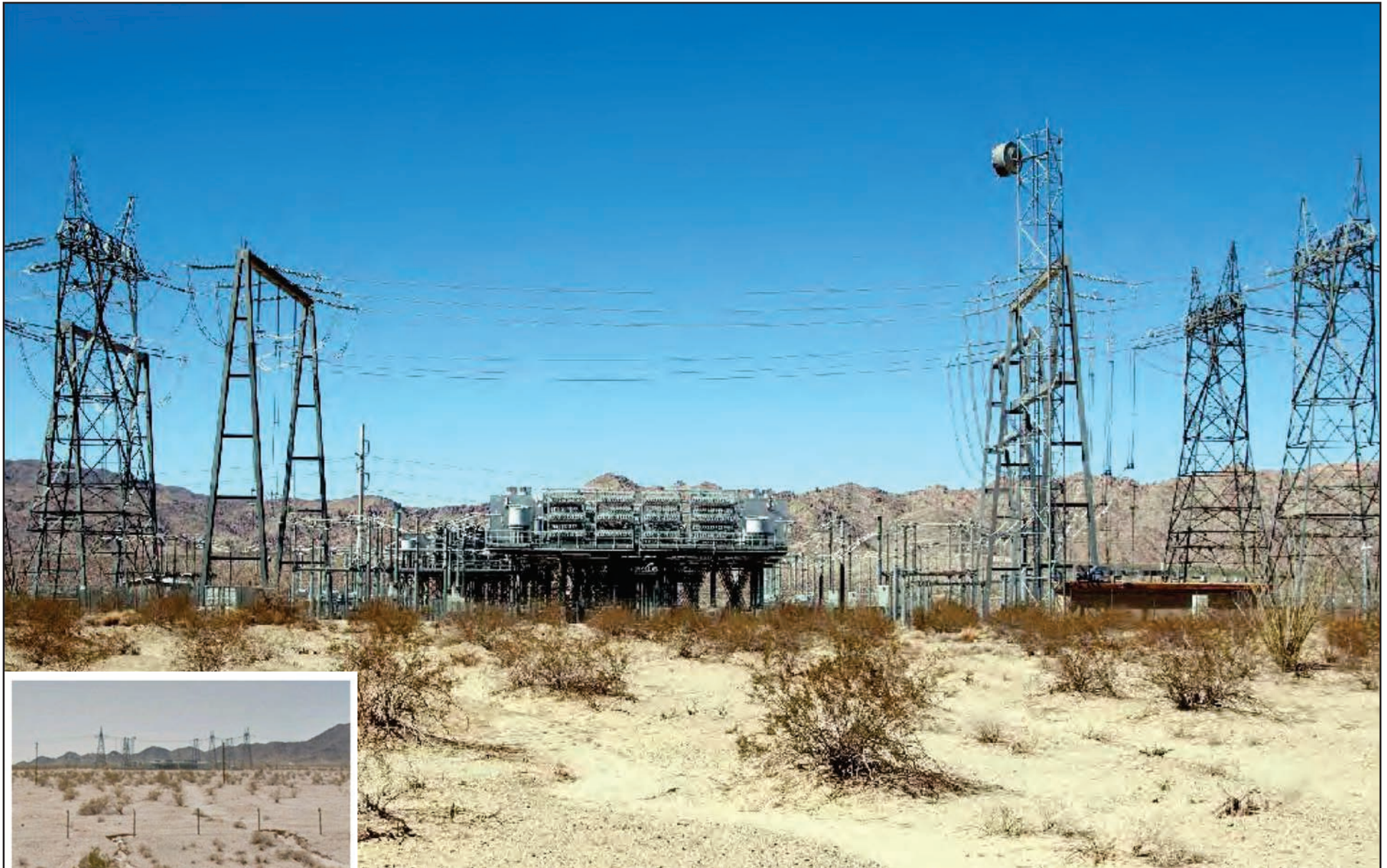
Figure 5.1-1 Devers-Red Bluff 500kV Mid-Line Capacitor
