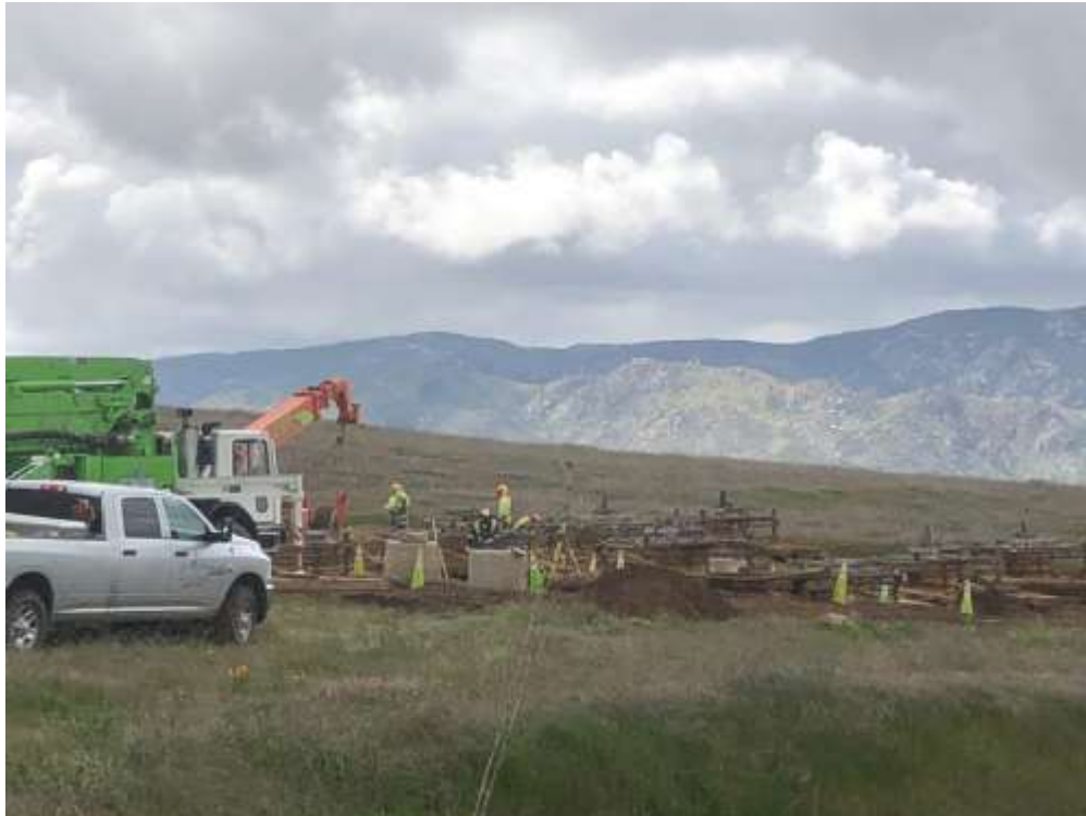
Photo 3 – Foundation Activities at Construction Area 4X07, Segment 4 (March 25, 2020).
