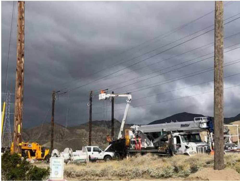
Photo 5 – Wire wreck-out activities at Construction Area 5X01, Segment 5 (March 25, 2020).
