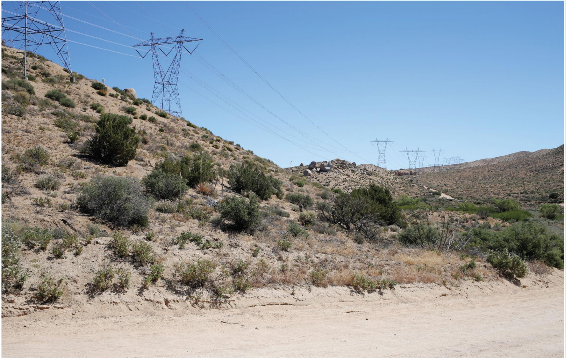
KOP 1: Existing view looking northeast from Bowen Ranch Road
