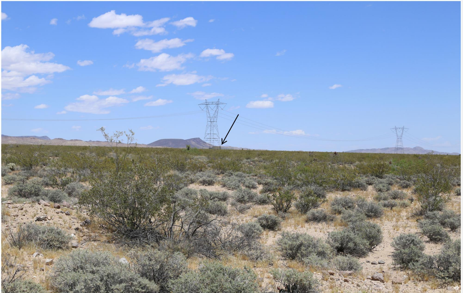
KOP 6: Visual simulation of the Proposed Project Lanfair Fiber Optic Repeater along the Lugo-Mohave 500 kV Transmission Line
