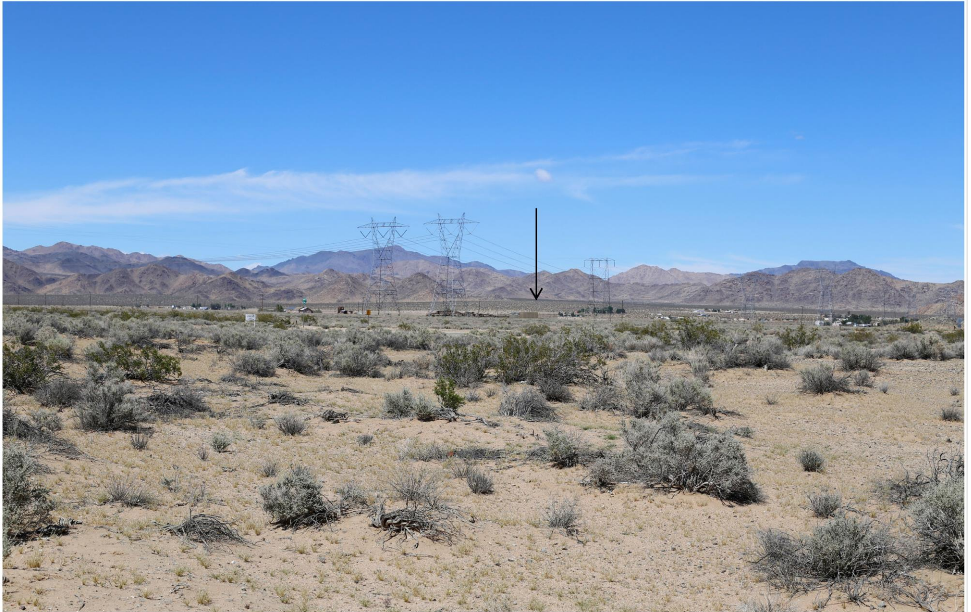
KOP 2: Visual simulation of the Proposed Project Barstow Fiber Optic Repeater Site along the Lugo-Mohave 500 kV Transmission Line
