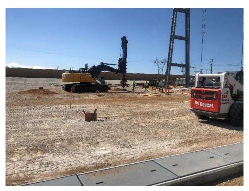
**Photo 1**: Drilling for foundations. March 13, 2021.
