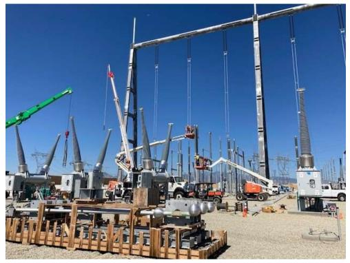
Photo 1: Installing bus supports at Lugo Substation (July 1, 2021).
